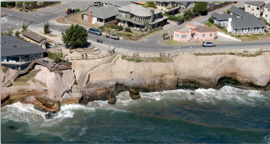
Figure 25. Photo depicting protection of visual resources and public access. A seawall visually blends in with the natural bluff while surfing access is also provided at Pleasure Point, Santa Cruz (2013). (Source: California Coastal Records Project )
