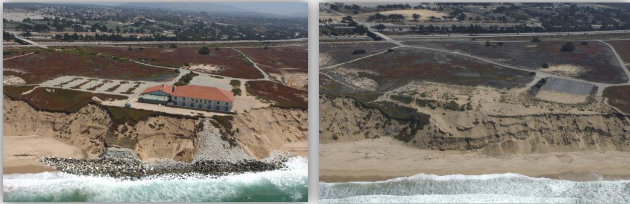
Figure 15. Photo depicting passive erosion. (Left) Passive erosion in front of a revetment at Fort Ord, illustrating the loss of beach where the development prevents the shoreline from migrating landward. The beach continues to migrate inland on either side of the revetment. (Right) Recovery of the beach following removal of the revetment and blufftop structure. (Source: California Coastal Records Project ).
