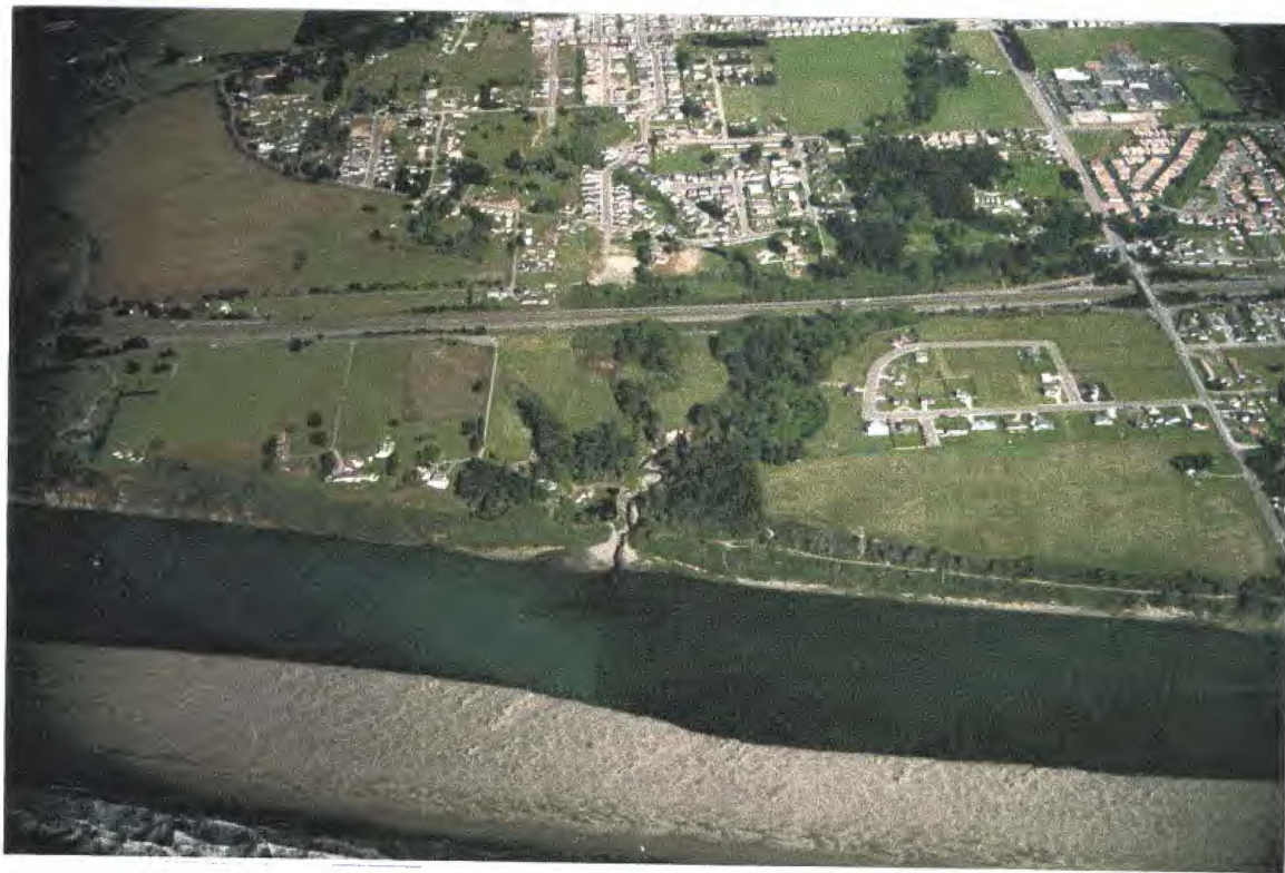
Erosion along east bank of The Mad River and Widow White Creek.
