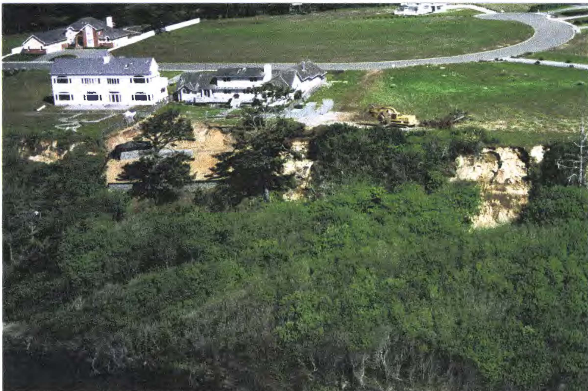
Bluff failure in back yards of Knotts Cove Subdivision. Undermining due to unstable soil.
