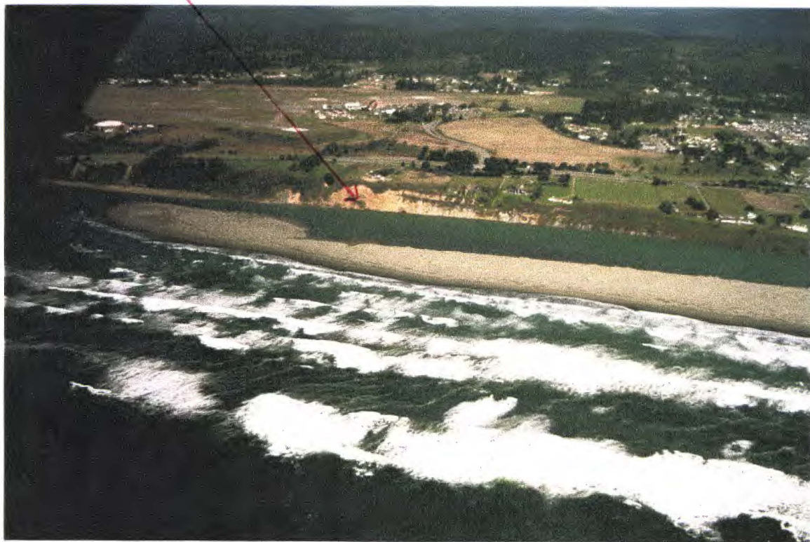
Bluff failure and seismic fault North of Sand Pointe Project.
