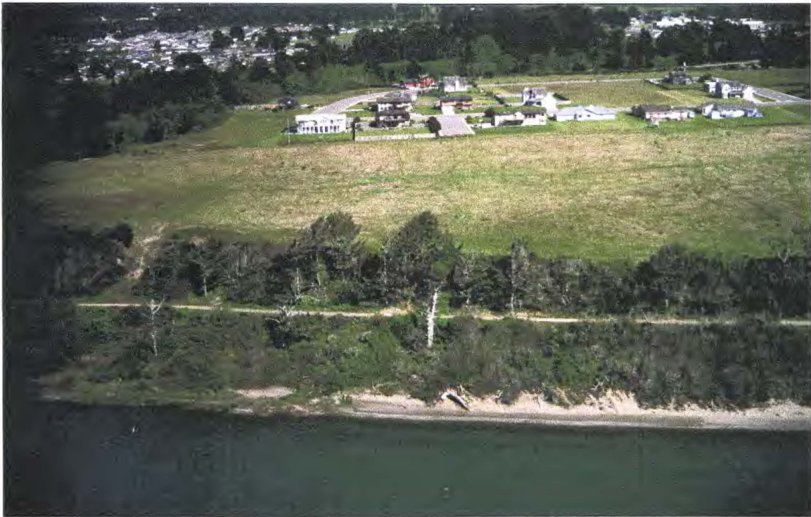
Visible erosion on Bluff above and below the Hammond Trail. You can see the water line, where the water was about two hour's earlier. The Hammond Trail is about 2/3 up the bluff. It is extremely hard to see but the Mad River Fault line can be seen at the low altitude oblique shots.
