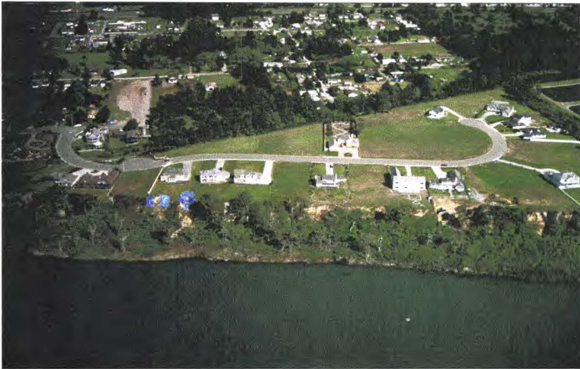
Erosion and bluff failure at Knotts Cove, one block south of Sand Pointe Project.
