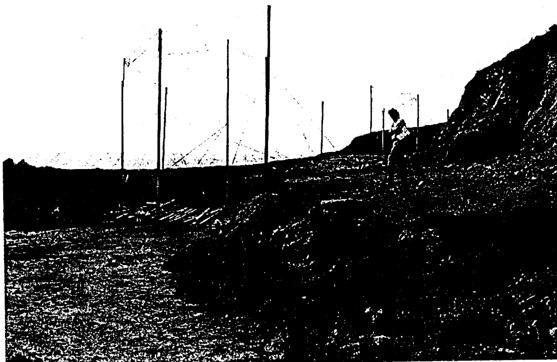
Photo 2. Project staking, looking north; theater/media area is staked at rightmost of photo (against bluff). Photo shows excavated building pad and cut face on right.
