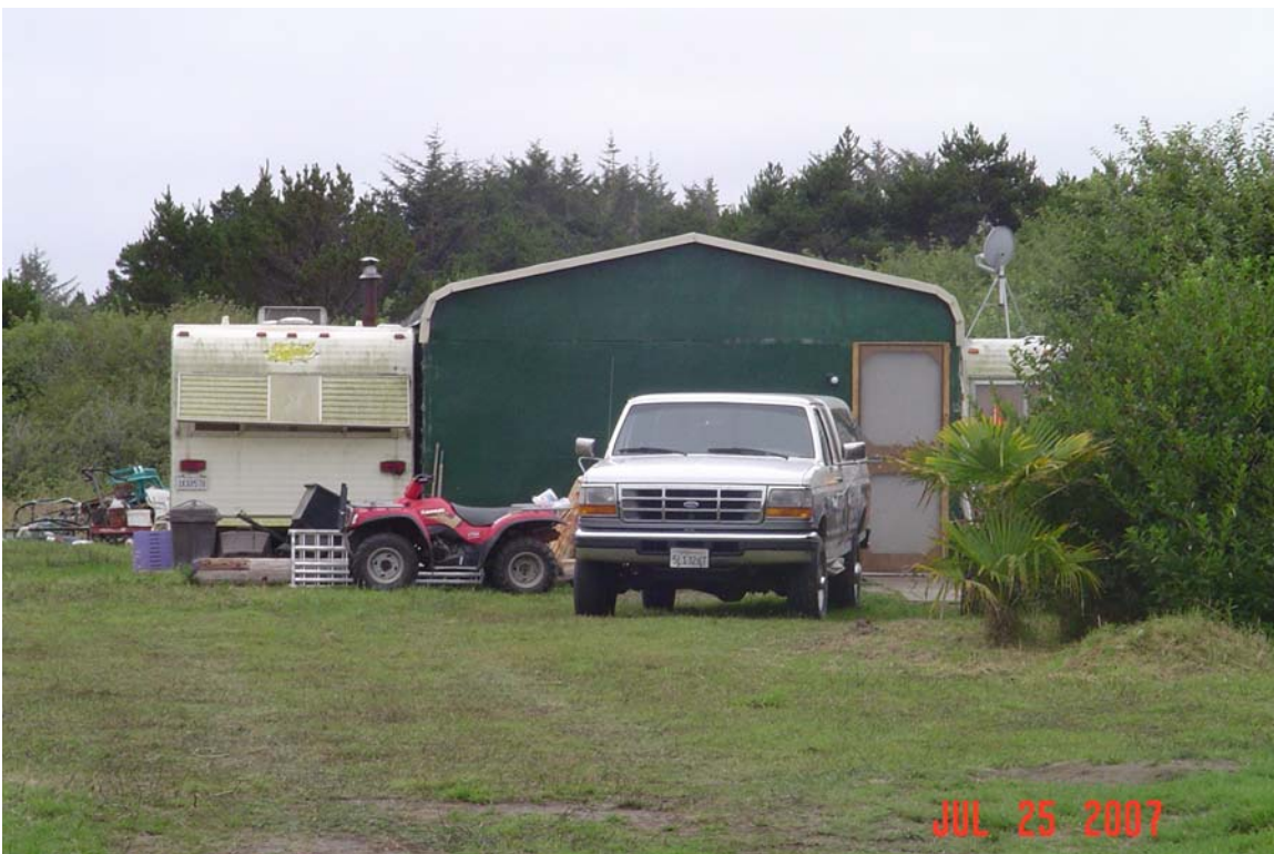
Exhibit 3g. July 25, 2007 photo of unpermitted structures, trailers, and vehicles on subject property.
