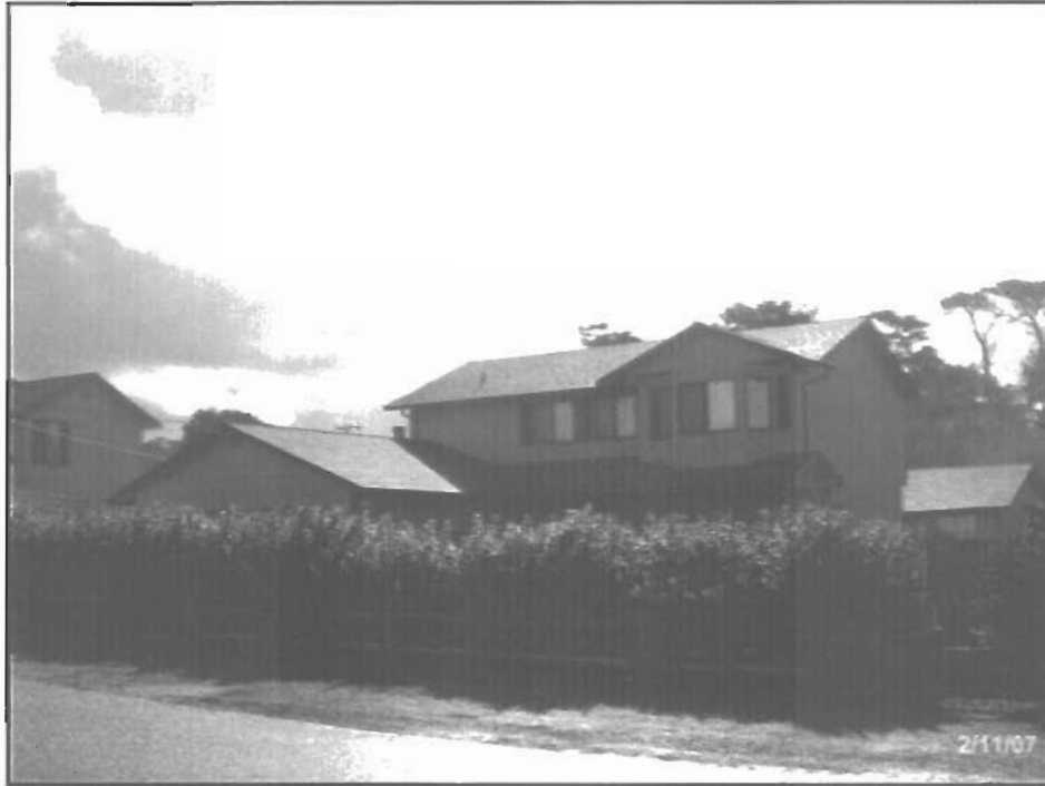
Photo 5. View of 814 Murray Road (next to 844 Murray Rd.) from the future Hammond Bypass Trail extension along Murray Rd. This is a two-story multi-family residential unit.
