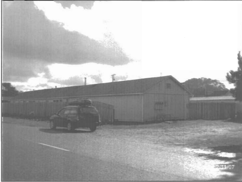
Photo 1. Multi-family residential unit on the corner of Murray Road and Daffodil Avenue, across the street from the subject parcel (view from the future Hammond Bypass Trail extension along Murray Rd).
