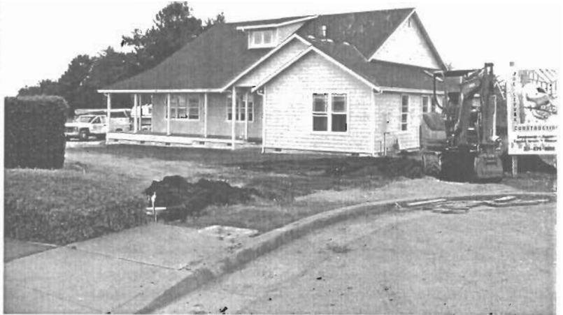
3000 Fortune Street (under construction)
