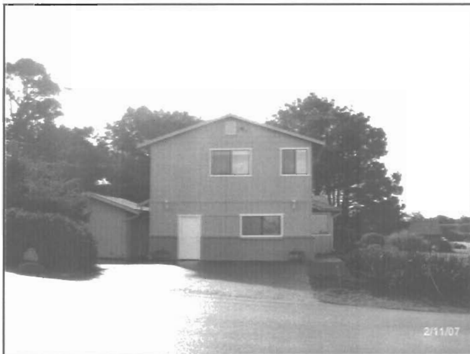
Photo 8. View of 2797 Kelly Avenue, next to 776 Murray Rd., from the future Hammond Bypass Trail extension along Murray Rd. This is a two-story single family residence approximately 2,100 square feet in size.
