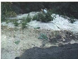
Slope with Drainpipe and Rock Rip-Rap at Pipe Outlet as **Energy Dissipator**
