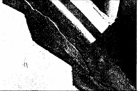
Photo 12. Concrete curb crack
