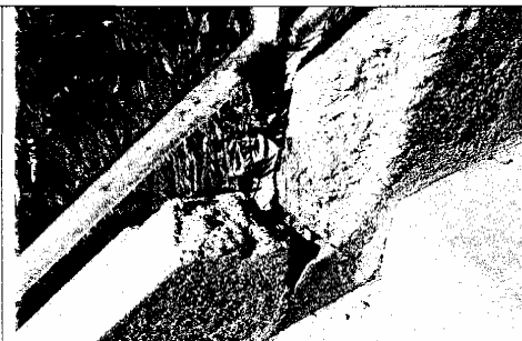
Photo 6. Guardrail anchor & curb failure
