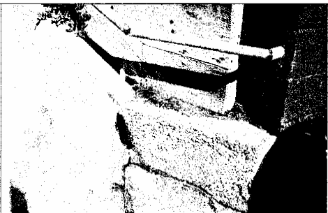
Photo 8. Guardrail anchored to wall
