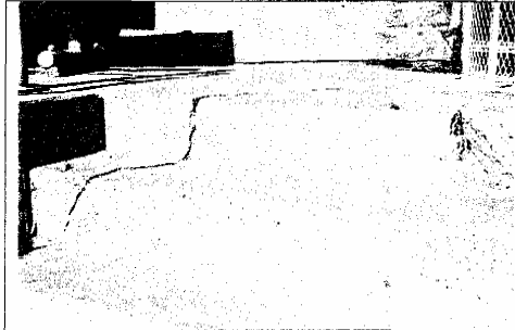
Photo 17. Concrete step cracks alkway and step cracks
