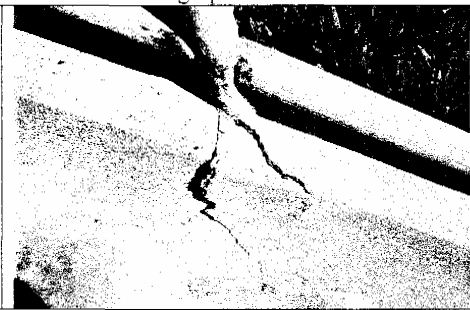
Photo 4. Guardrail anchor & curb failure
