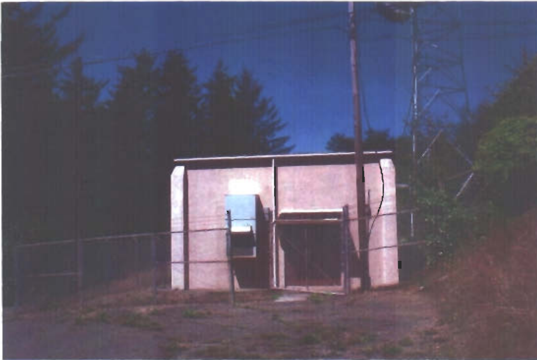
1. Looking Northward at the existing Verizon telecom bldg. and tower structure.
