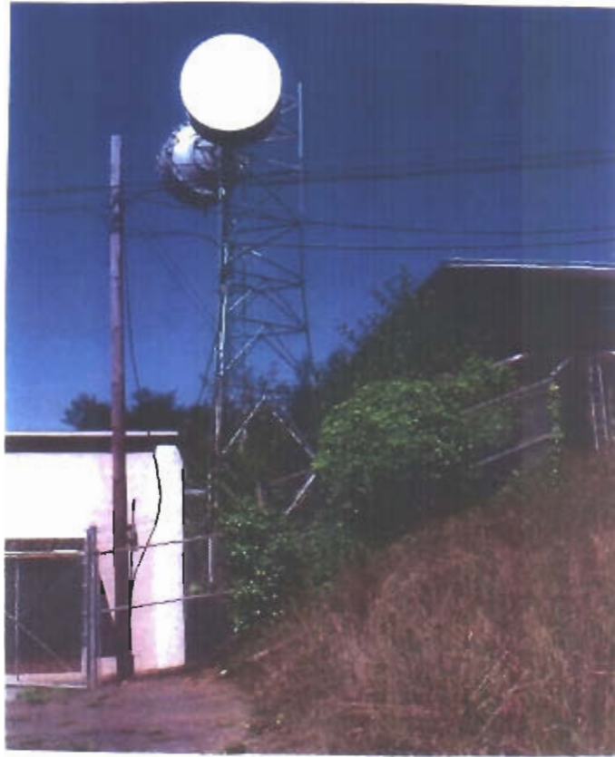
3. Looking Northward at the existing Verizon tower structure with antennas.
