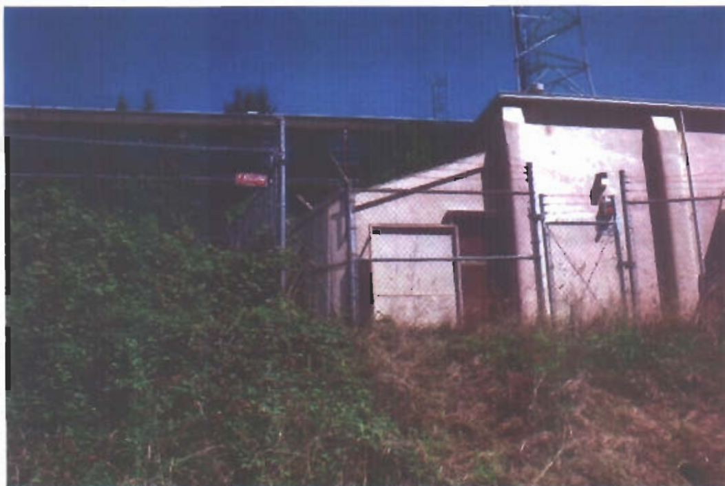
5. Looking Eastward at the Verizon telecom bldg. and tower structure behind it.
