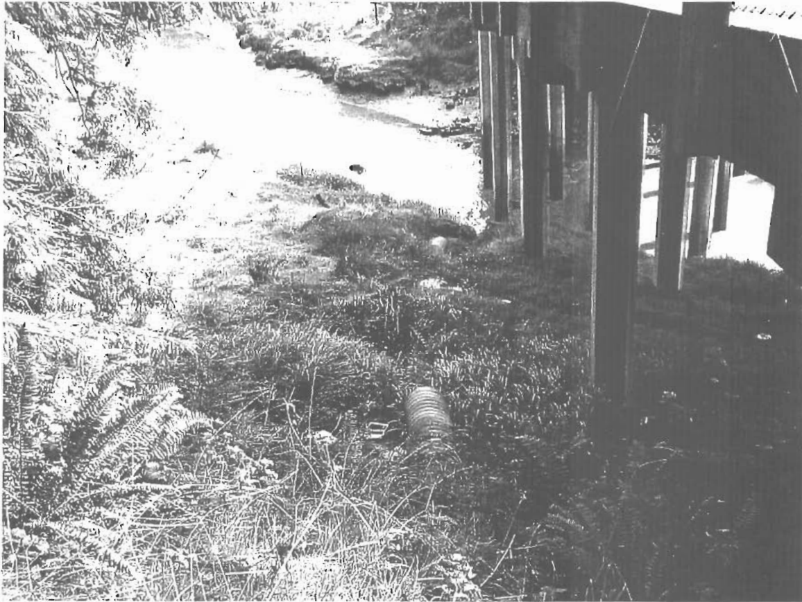
Photo #2: Shows lower drain pipe to be removed. Rock is to be placed within eroded bank.
