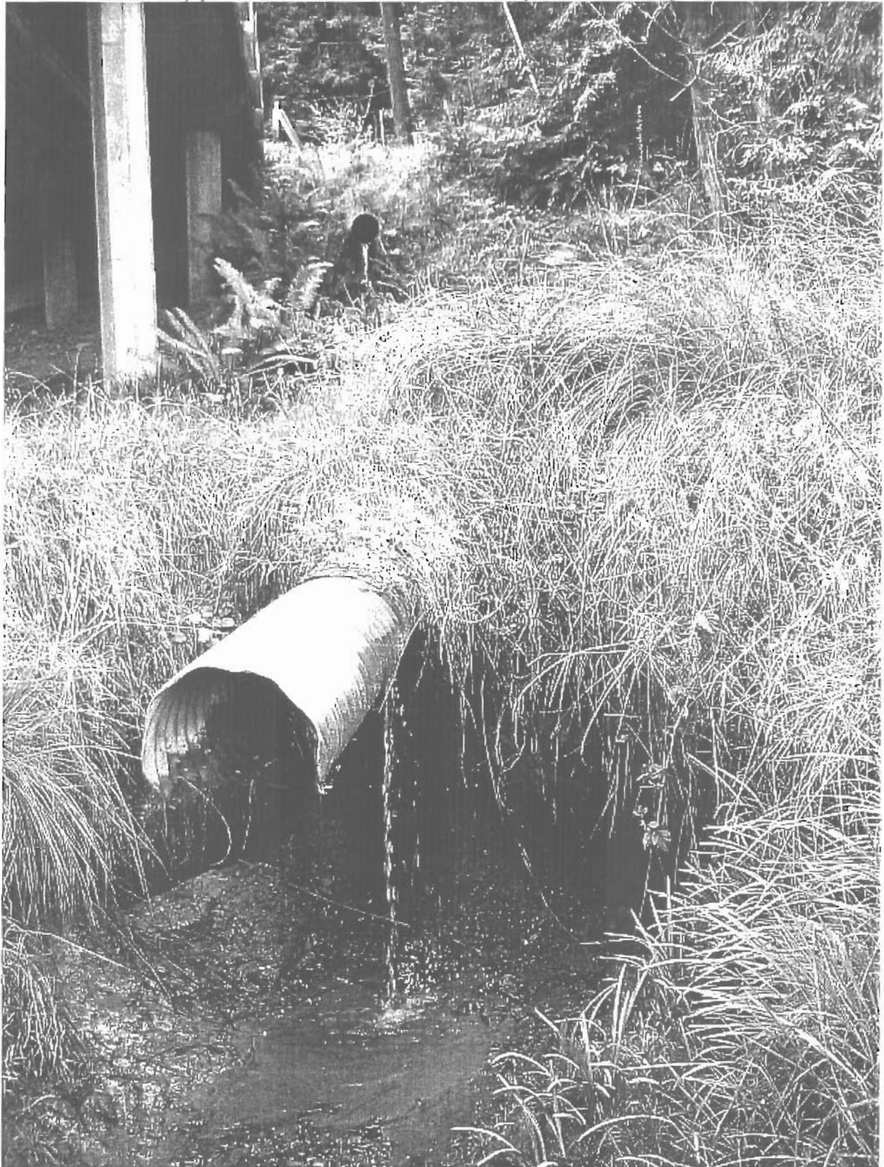
Photo #3: Shows both outfalls. Upper outfall will be replaced and rock dissipater will be placed below new outfall. Lower outfall pipe to be removed and eroded bank to be protected with large rock.
