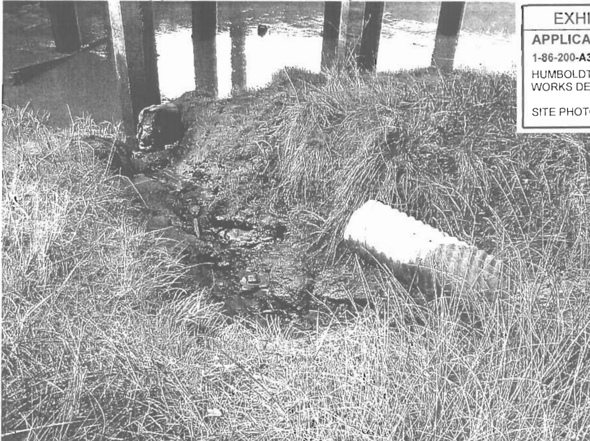
Photo #2: Shows lower drain pipe to be removed. Rock is to be placed within eroded bank.
