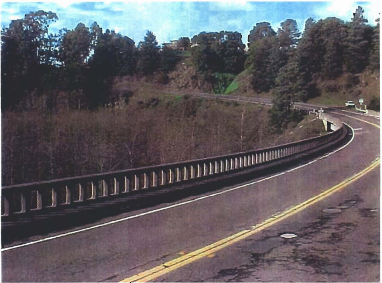
Existing rail on Greenwood Creek Bridge, looking north.
