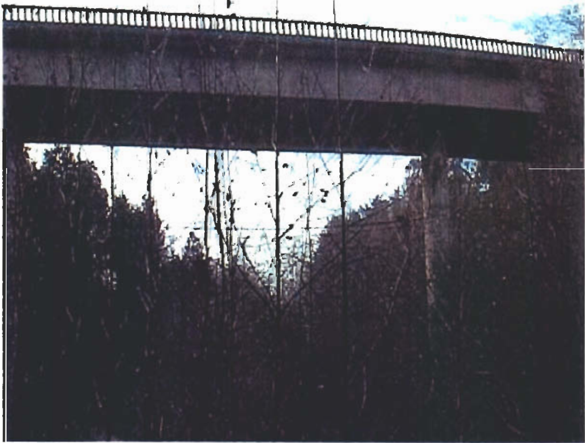
Looking upward towards existing Greenwood Creek Bridge from the east.
