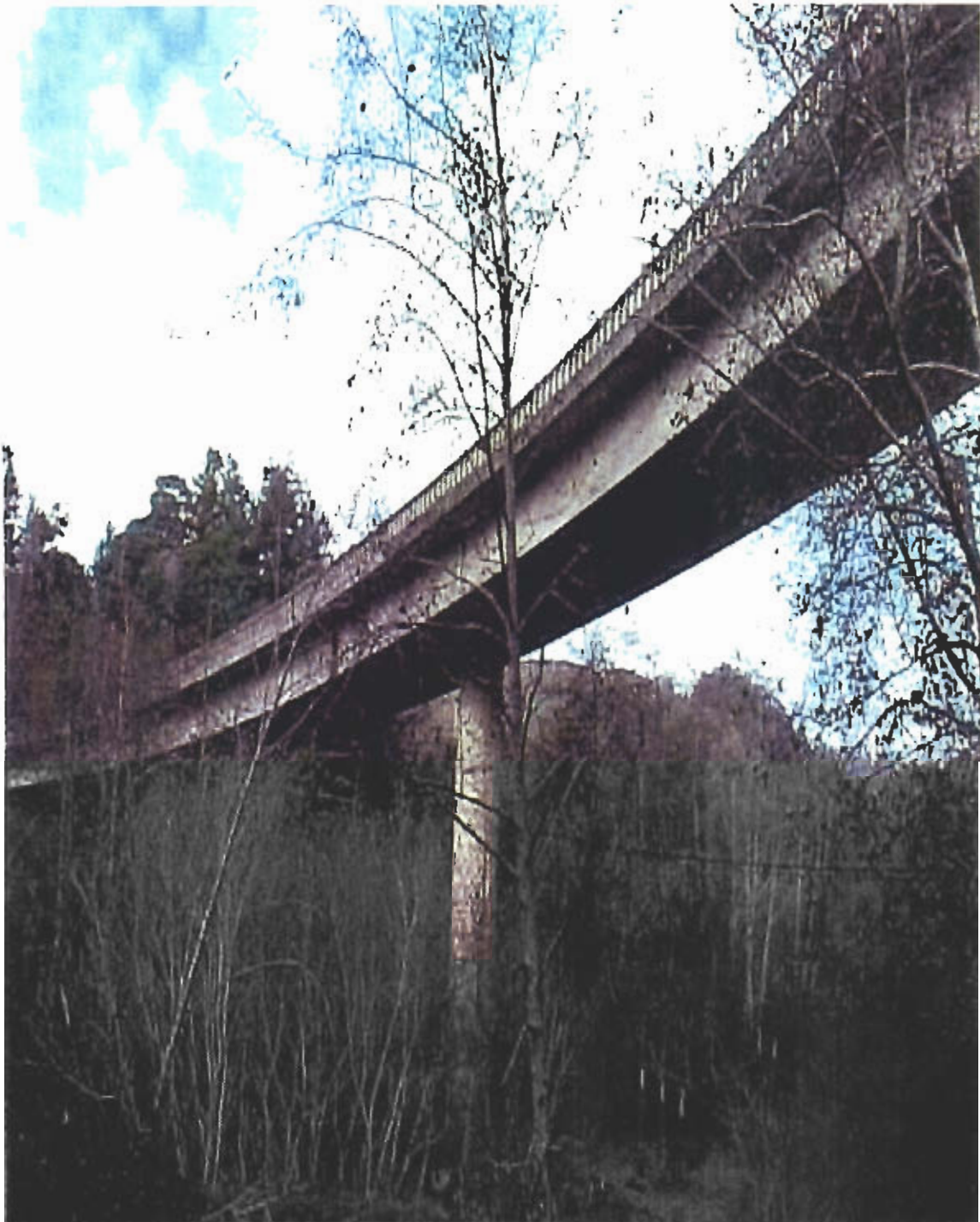
Looking north-east to existing Greenwood Creek Bridge.
