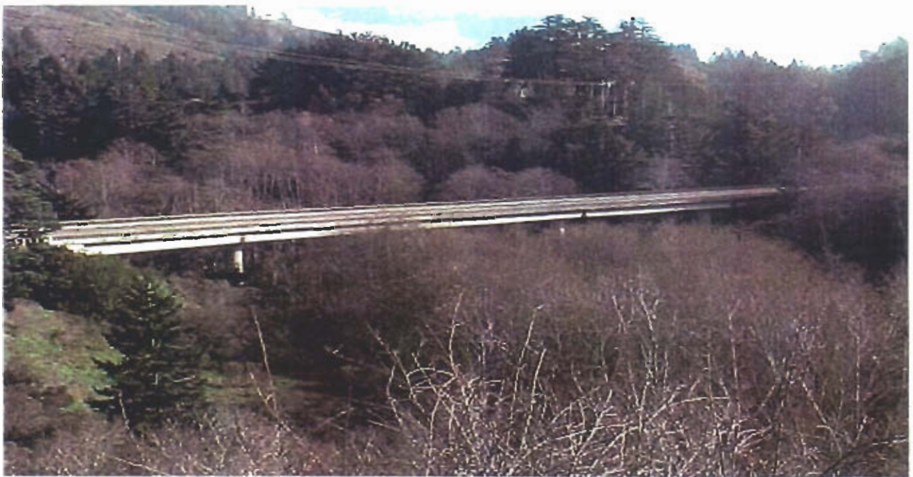
Looking south-east towards existing Greenwood Creek Bridge.
