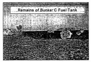
Bunker C oil was the primary fuel used for locomotives at the site until 1954. After 1954, diesel fuel was used for locomotives. During site operations, Bunker C oil was stored in a 650,000-gallon aboveground tank. In 1954, the top of the large Bunker C fuel tank was removed to make a secondary containment structure for two 12,700-gallon diesel fuel tanks. Fuel storage at the site was discontinued in 1984 as site operations decreased and a tank truck was used to fuel locomotives.
