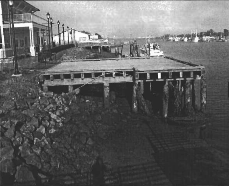
Photo 9: View west of the existing eastern wooden wharf proposed for demolition (taken August 1, 2007).
