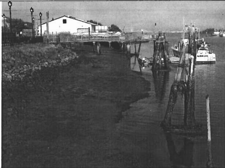
Photo 1: View west facing the existing dock and pier structure serving the California Department of Fish and Game (CDFG) at the foot of J Street (taken August 1, 2007).
