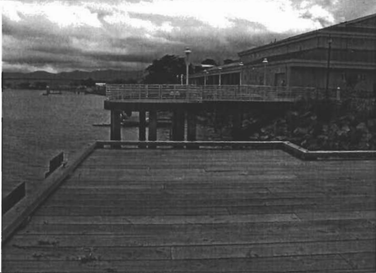
Photo 8: View east from the existing eastern wooden wharf proposed for demolition (July 18, 2007).
