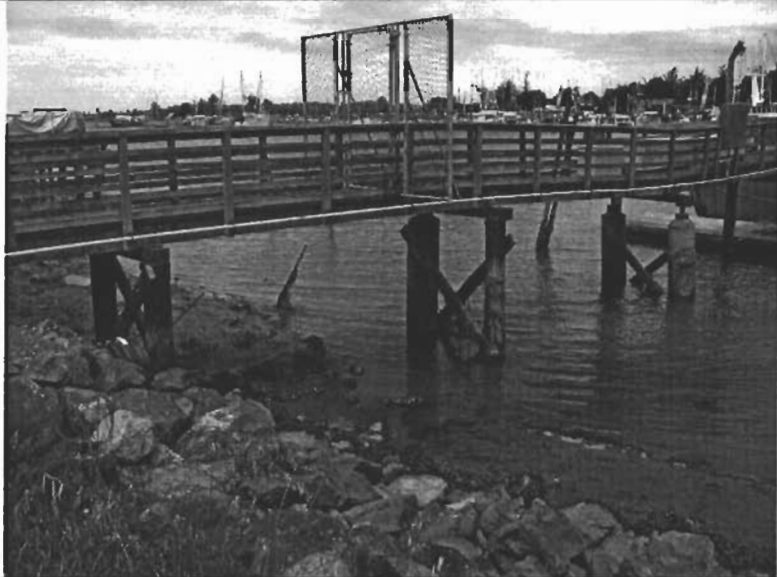
Photo 2: Close-up of existing dock and pier structure serving the CDFG at the foot of J Street. The red arrow is pointing towards an existing outfall pipe immediately to the east (taken July 18, 2007).
