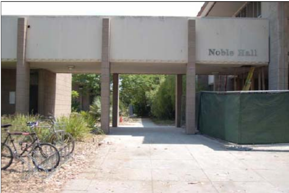
Corridor 21: View looking east along the pedestrian pathway located through Noble Hall.
