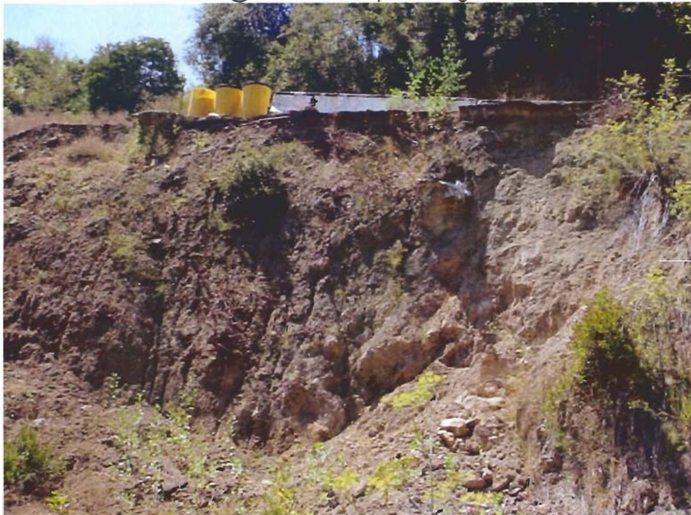
@ MM 4.98 close view of the slope sliding
