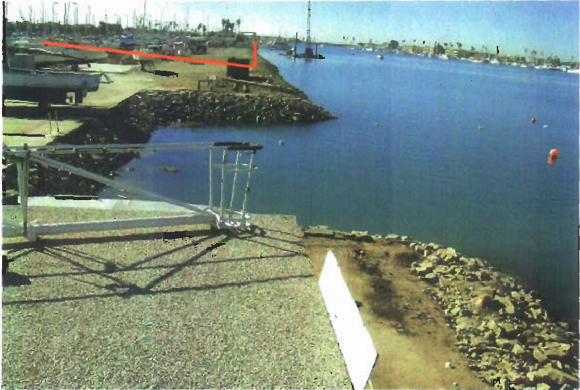
Looking south from boatyard building toward the proposed pedestrian pathway and the travel lift pier area. Any pathway would have to turn east into the boatyard area at orange line.
