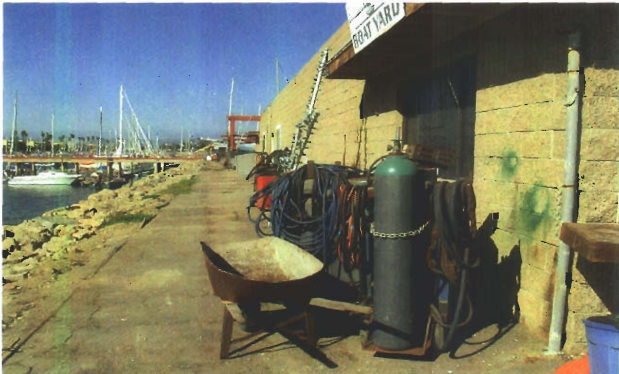
Area on the waterside of the boatyard building with insufficient room for pedestrian pathway.
