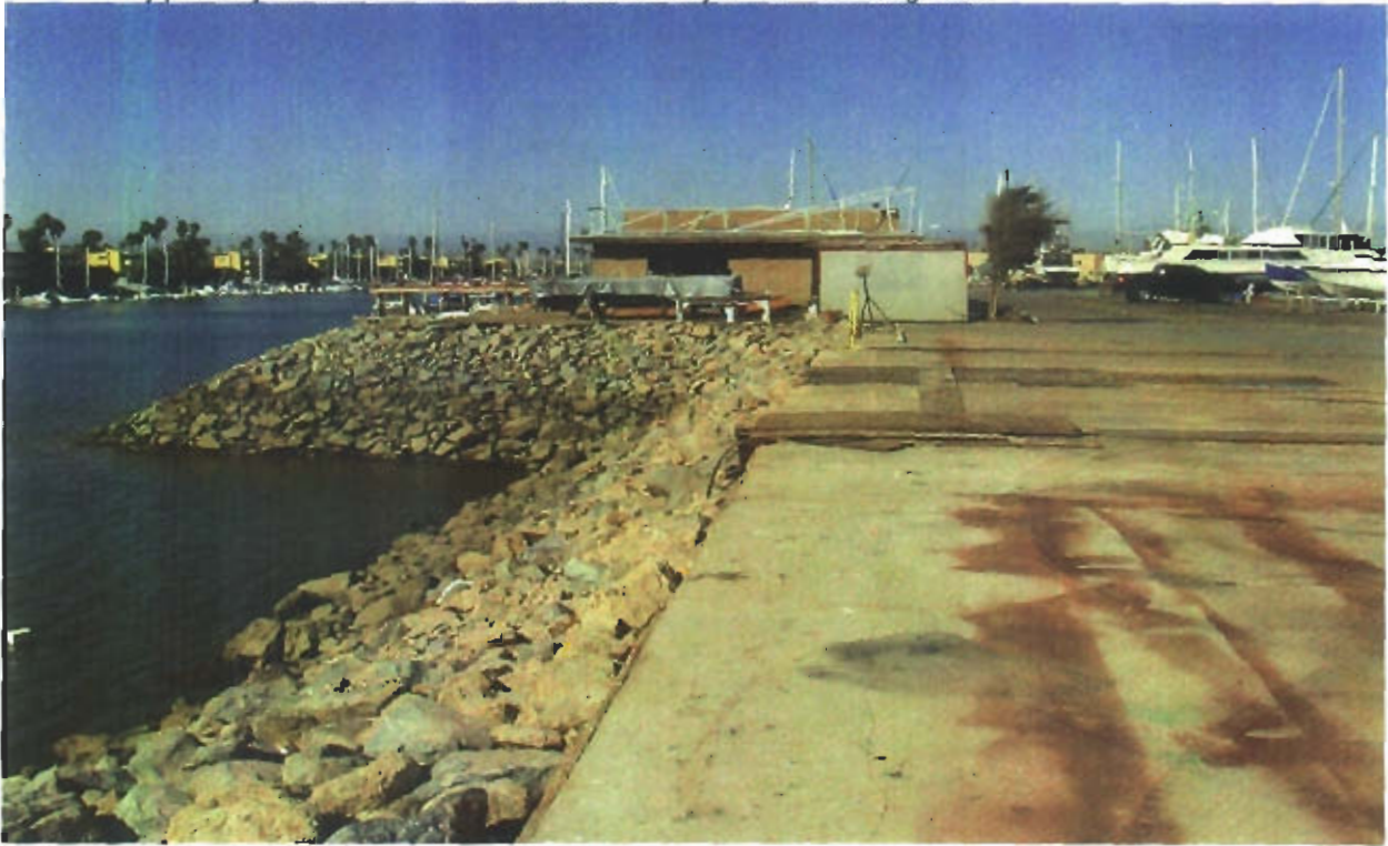
Looking north across travel lift ways into boatyard.
