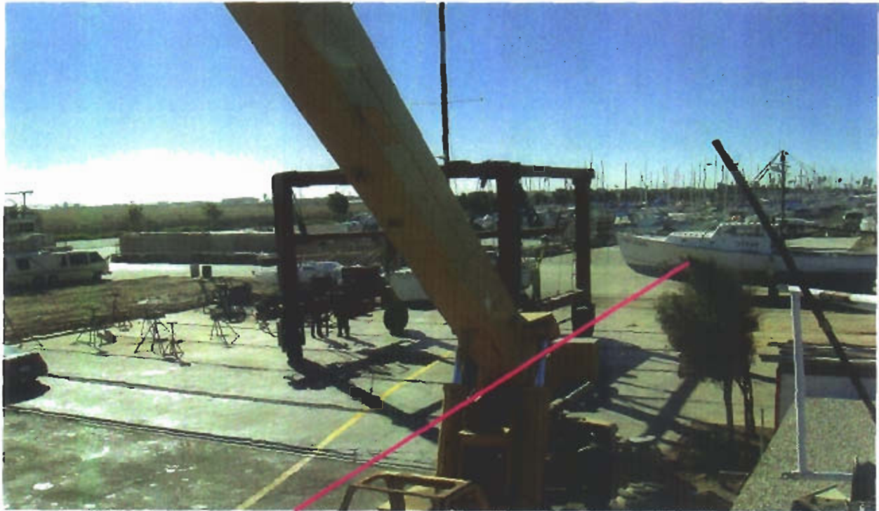
Boatyard activities that present a public safety hazard to public walking through boatyard. Pink line shows path that pedestrians would have to travel to get through the boatyard.
