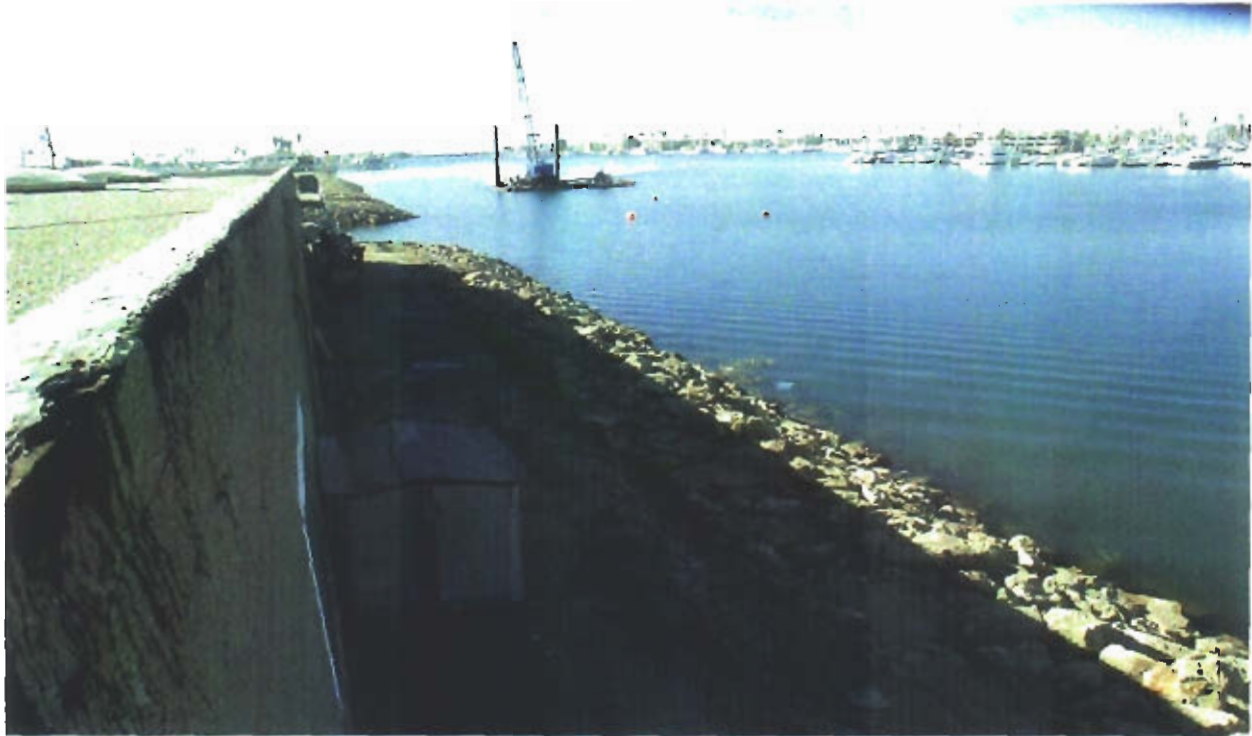
Area on the waterside of the boatyard building with insufficient room for pedestrian pathway.
