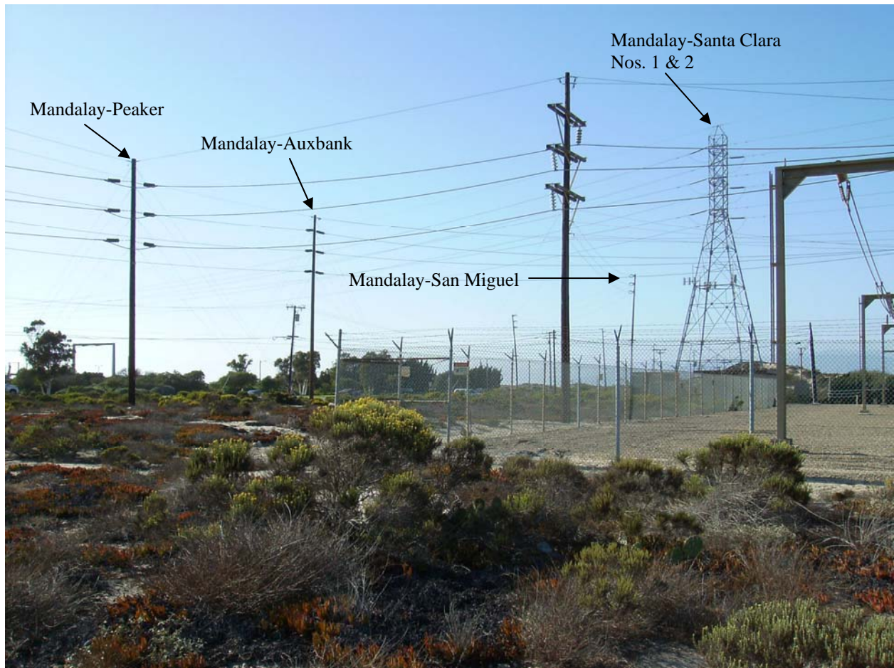
Figure 8. Looking northwest from Mandalay Substation. Mandalay-Peaker 66kv line and Mandalay-Auxbank 66kv line exit the substation westward and cross Harbor Blvd. Mandalay-San Miguel 66kv line heads northward. Mandalay-Santa Clara Nos. 1 & 2 220kv lines run on lattice steel towers from Reliant Mandalay Generating Station to Santa Clara Substation in the east (bypassing the Mandalay Substation).
