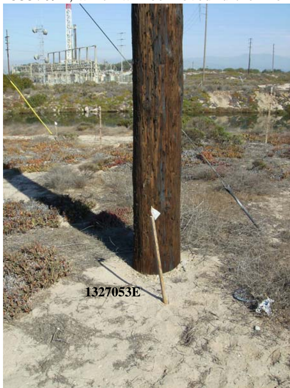
Above: Figures 17 and 18. New taller pole 4533708E will be placed in the staked location shown. Existing pole 1824140E, to be removed, is seen in the background of Figure 17. Below: Figures 19 and 20. Existing pole 1327053E will be replaced by new taller pole 4533709E, which will be moved further from the Mandalay Canal in background.
