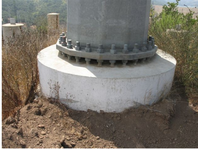
Figure 11. Typical TSP base and foundation.
