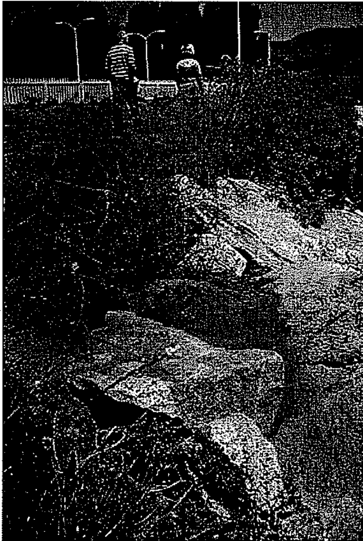
Figure 14. Failing loose boulder riprap placed by Mariposa Land Co. on Malibu Creek. North facing picture taken on June 22, 2009.
