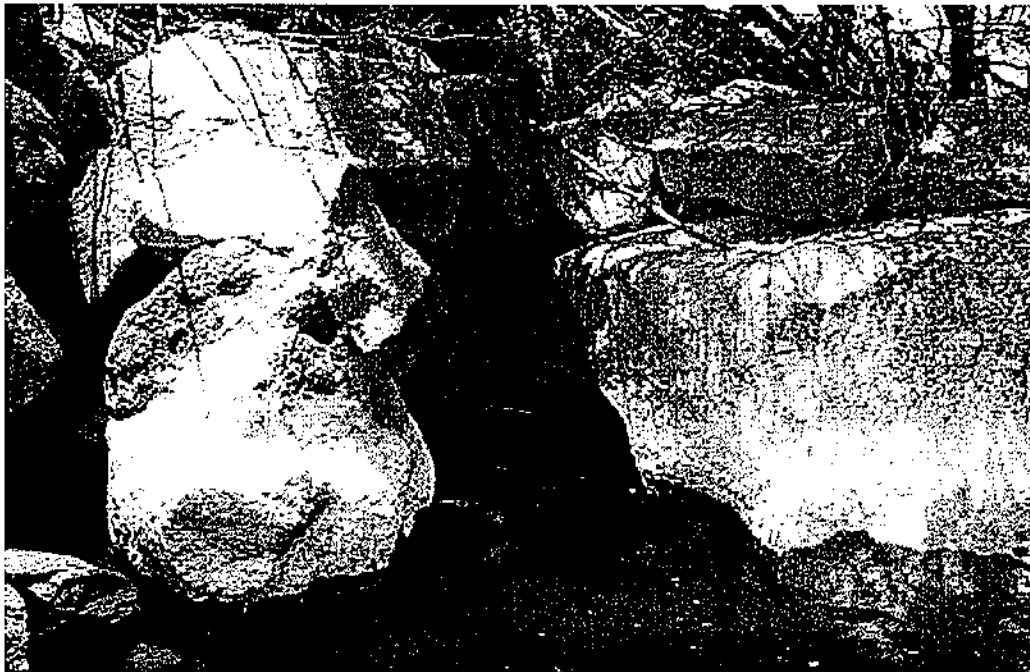
Figure 13. Failing loose boulder riprap placed by Mariposa Land Co. West facing picture taken from Malibu Creek on June 22, 2009.
