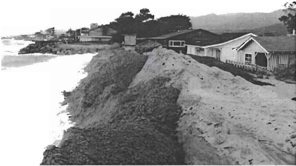
In some years the berm requires maintenance. In this photo, new sediment has been pushed up to the remaining berm to fend off another high tide.
