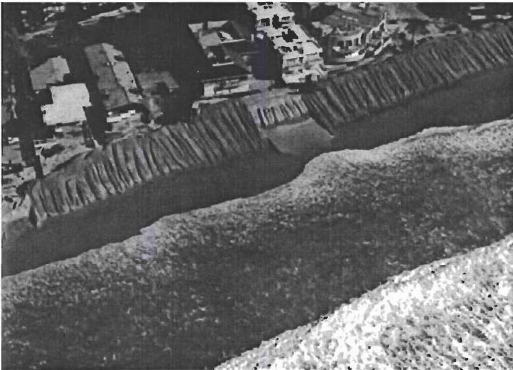
Aerial view of berm in the Holly Avenue to Elm Avenue block; this picture was taken during reconstruction after a major erosion event.
