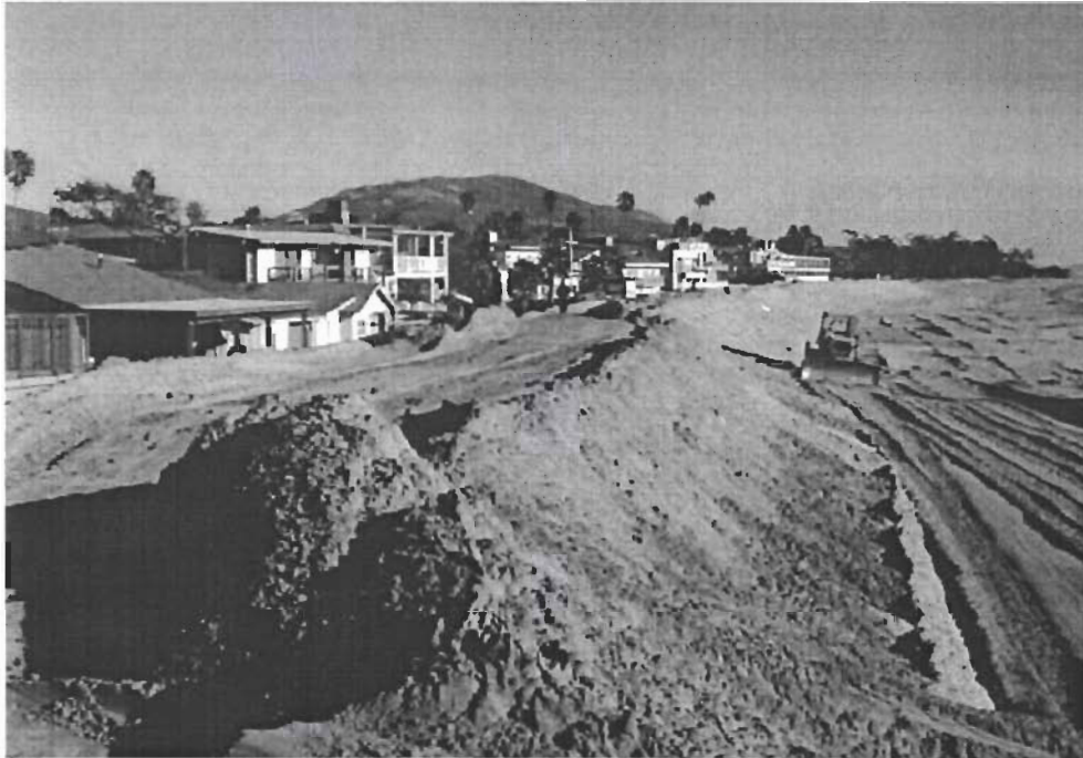
View from Ash Avenue looking east taken November 2008 – Berm just completed for 2008/2009 winter; note wide berm top allowing pedestrian parallel access to coastline
