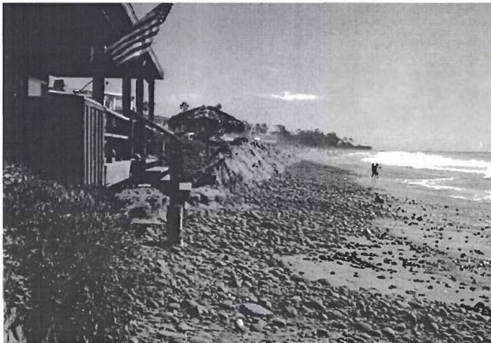
View from Ash Avenue looking east taken February 2003 – Berm has completely washed out after high tide; USGS study suggests end effects of Sandyland Cove seawall contributes to acute erosion problem at this location
