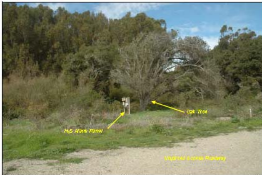
Photograph 37. H 2 S alarm panel in proximity to the unpaved access roadway paralleling the western boundary of the Venoco Ellwood Onshore Facility.
