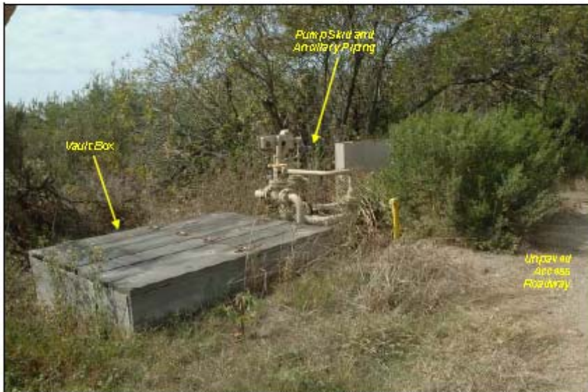
Photograph 36. Ancillary equipment and wooden valve box at southern termination of Bell Creek O-3 pipeline segment.
