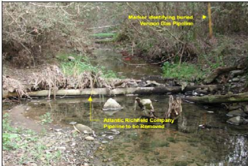
Photograph 27. View looking north showing exposure of O-3 Pipeline Segment across Tecolote Creek (photo taken in Summer 2004).
