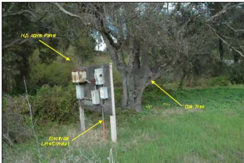
Photograph 38. H 2 S alarm panel and electrical line/conduit.
