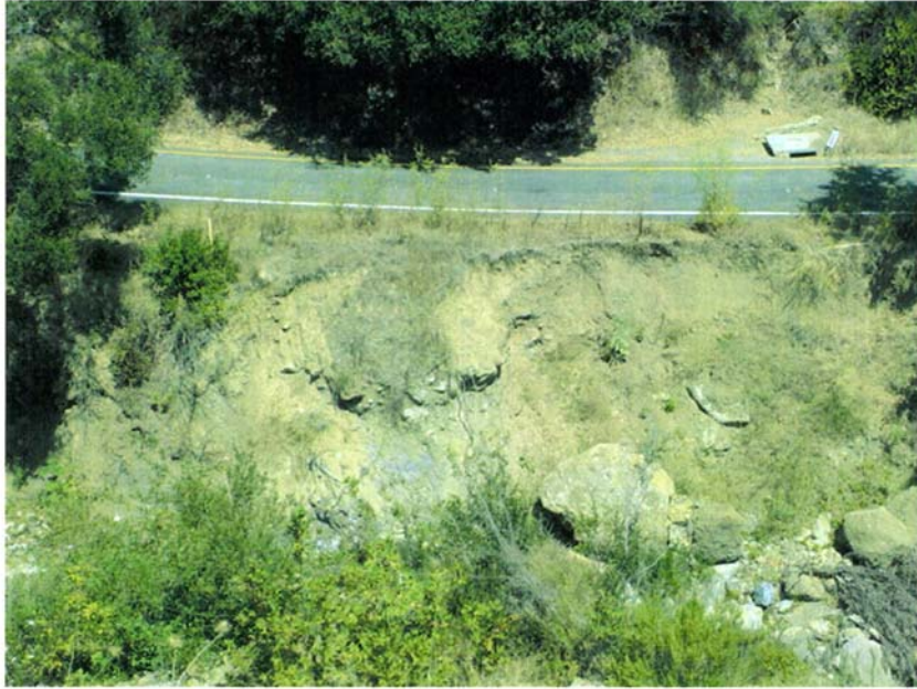
Aerial view @ MM 5.04 of slope failure
