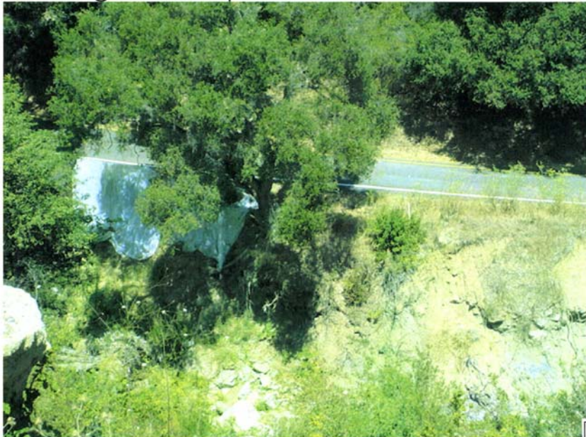
SW Aerial view @ MM 5.04 of slope failure.
