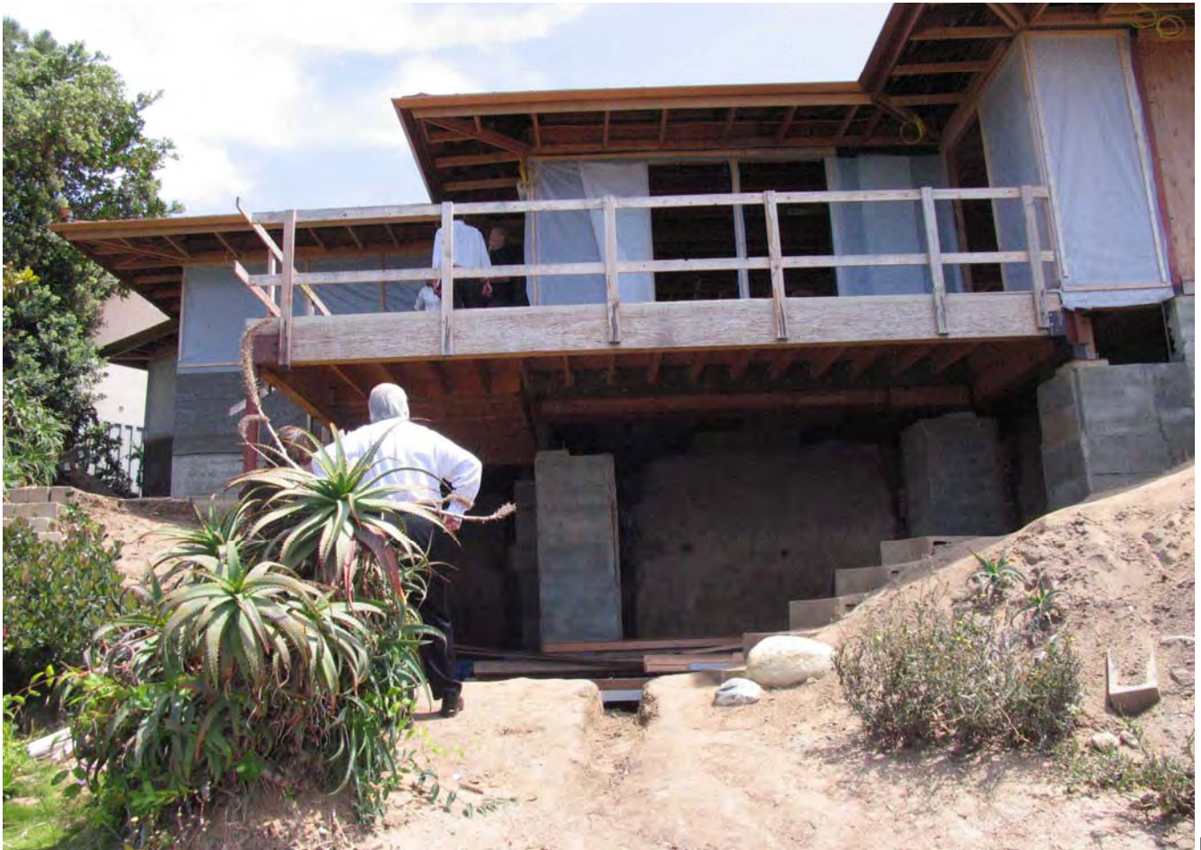
STAFF PHOTOGRAPHS OF SITE ON 6/2/2010
