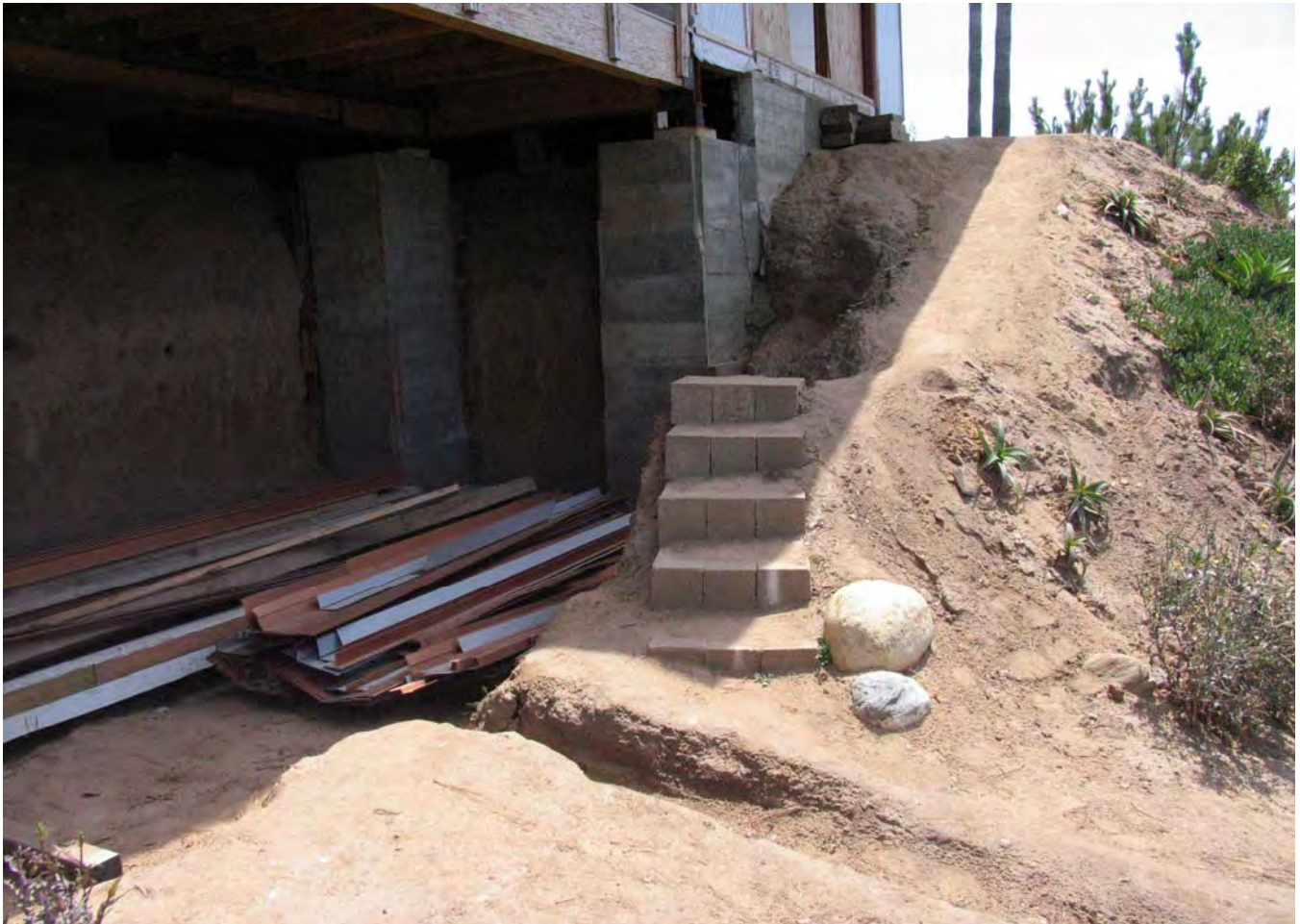
STAFF PHOTOGRAPHS OF SITE ON 6/2/2010
