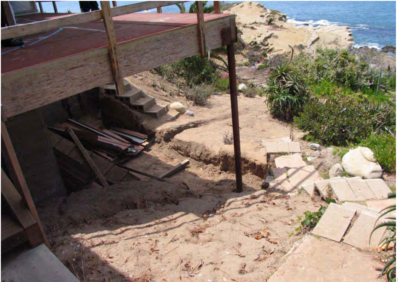
STAFF PHOTOGRAPHS OF SITE ON 6/2/2010
