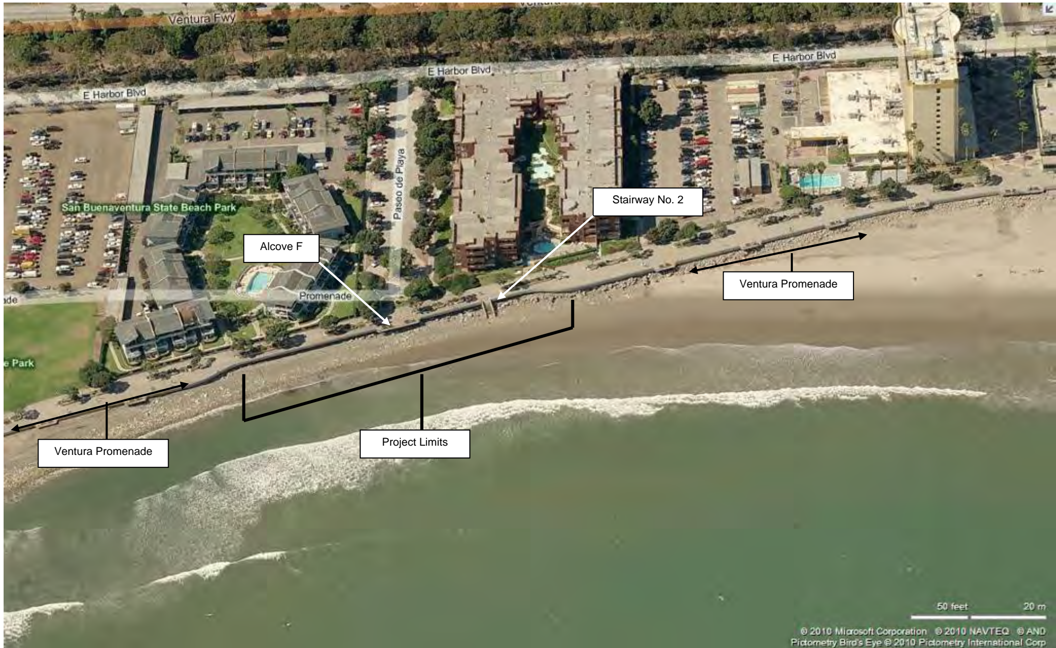
Exhibit No. 2b CDP 4-10-001 Project Aerials
