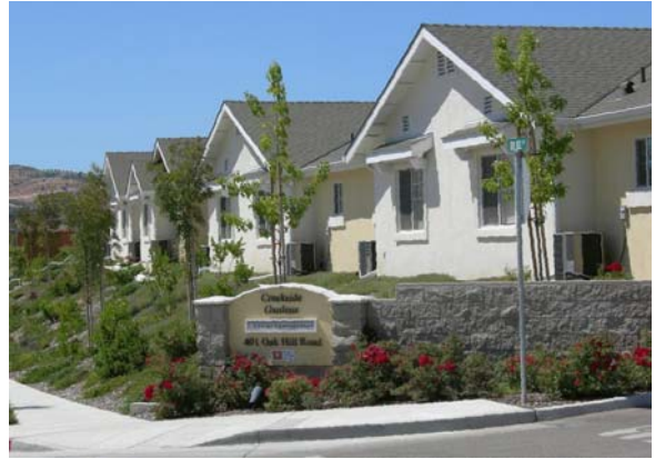
Figure 1-10: Creekside Gardens affordable housing
