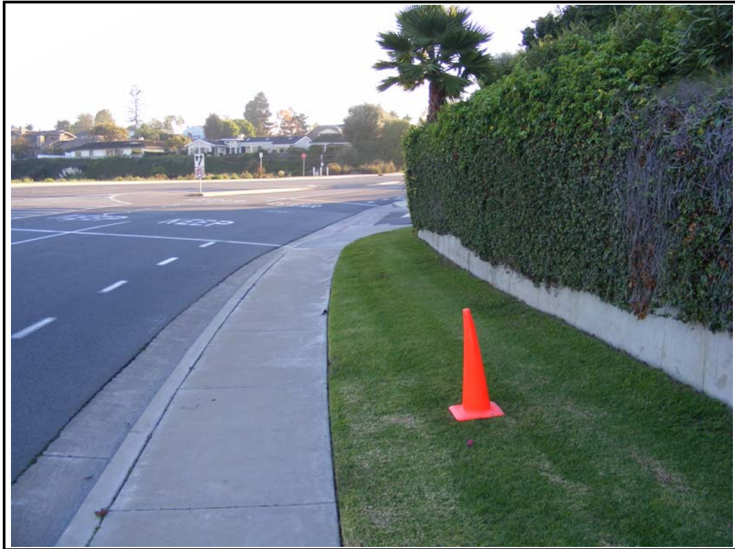
VIEW OF APPROXIMATE LOCATION OF METER PEDESTAL, ±91 FEET N FROM C/L PRIVATE ROAD, ±9 FEET W OF CONCRETE ROAD EDGE
