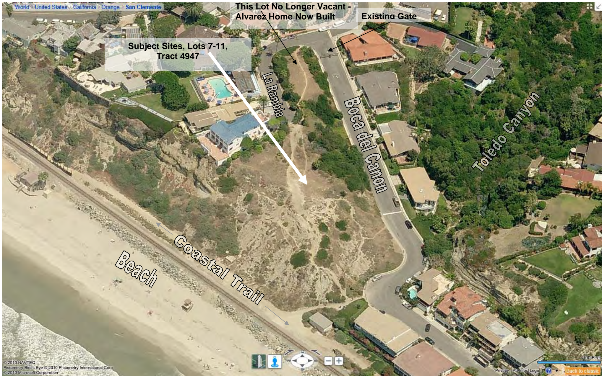
Oblique Aerial View of the Nine Vacant Lots, Including the Subject Sites, Lots 7-11
