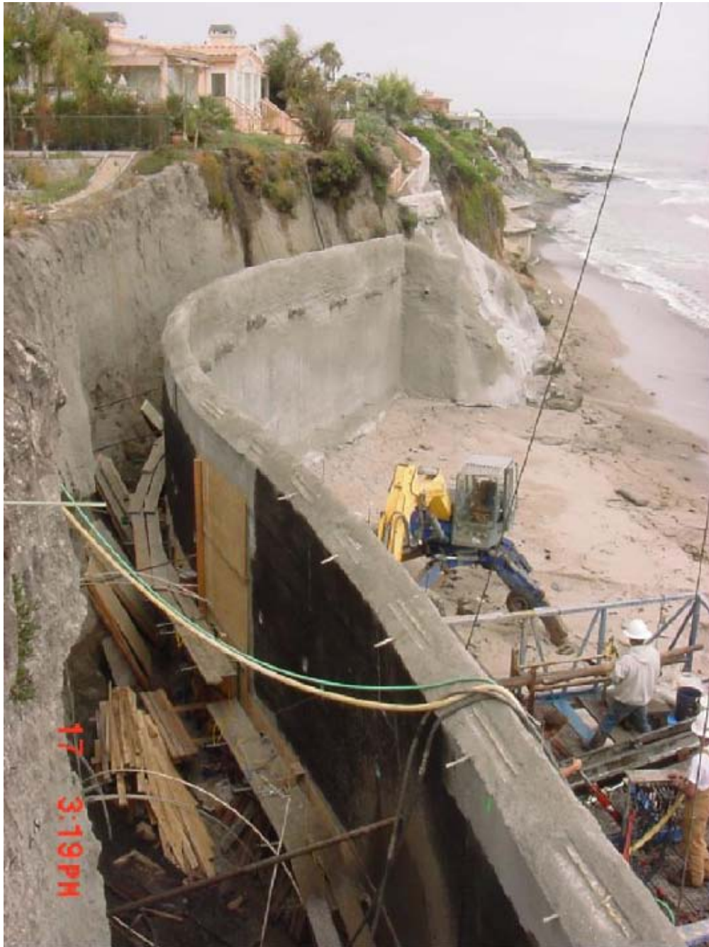
Figure 2-18 Sculpted Concrete/Shotcrete Wall at Florin Street in Pismo Beach
