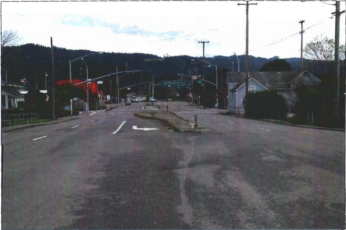
Photograph No. 1: Western Project Area – View East from I Street
