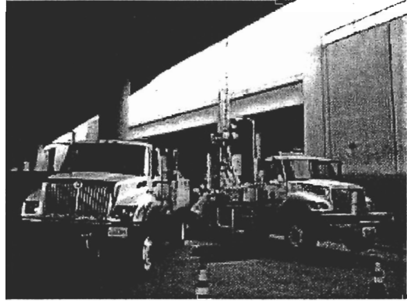
Photo 2. Onshore drilling operation.
