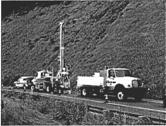
Photo 1. Onshore drilling operation.
