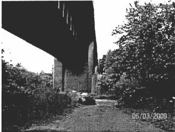
Photo 13. Access road facing North.
