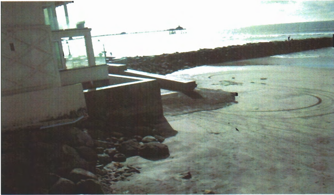
Photo 1 - Taken January 1, 2010 of Palm Ave access ramp from balcony 682 Ocean Lane
