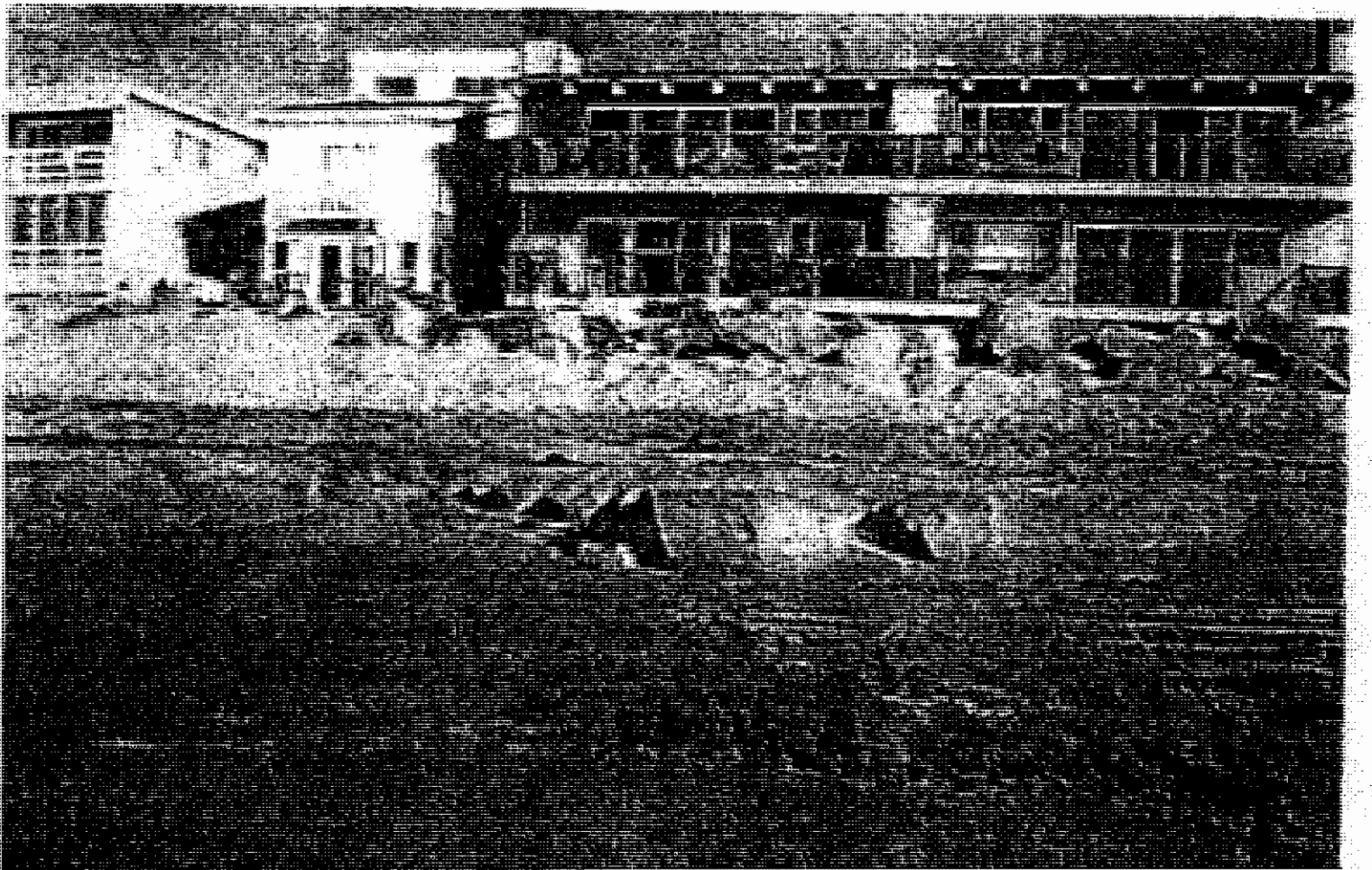
PHOTO 1: Looking north along revetment alignment, March 2010. Note that the revetment crown was originally situated at the floor level of the balcony to the right.
