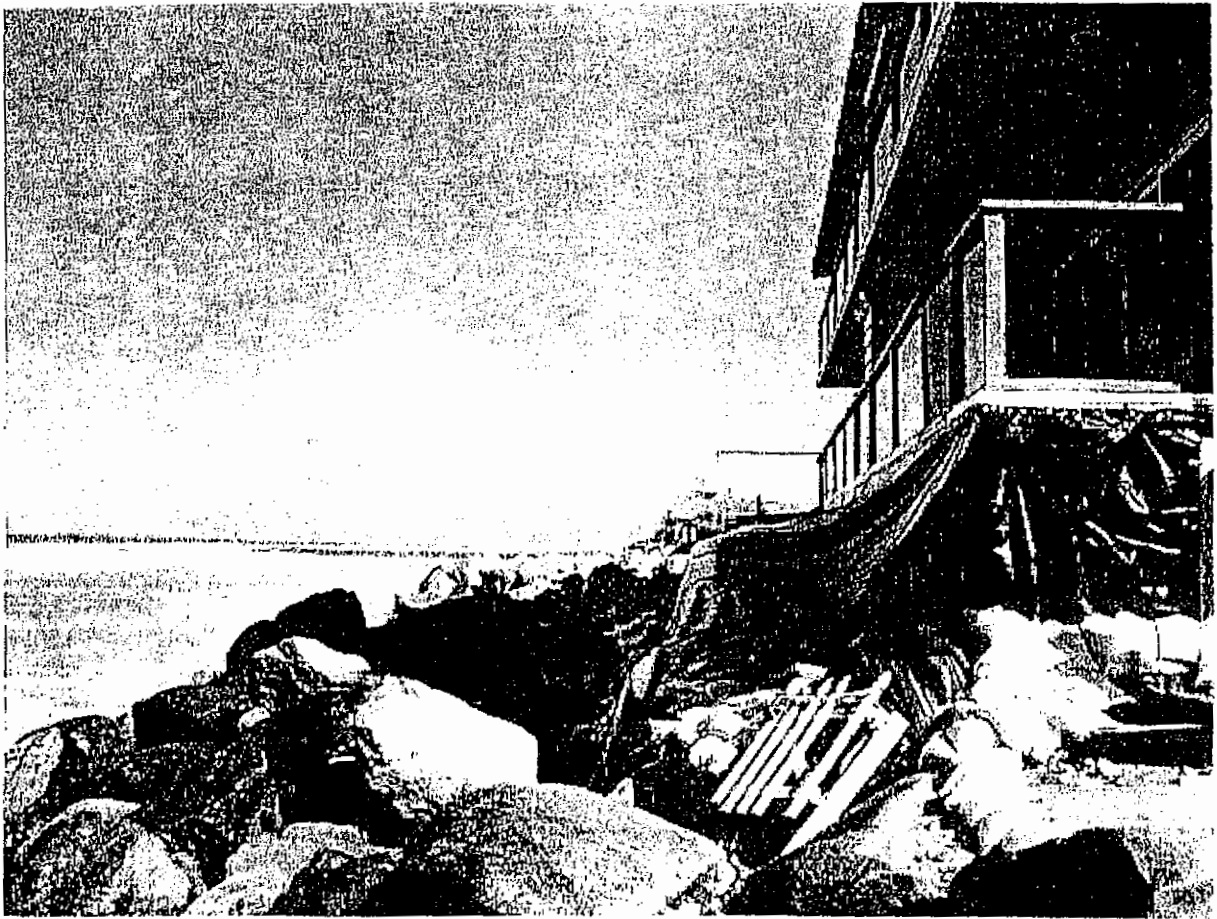
PHOTO 1: Looking north along revetment alignment, March 2010. Note that the revetment crown was originally situated at the floor level of the balcony to the right.
