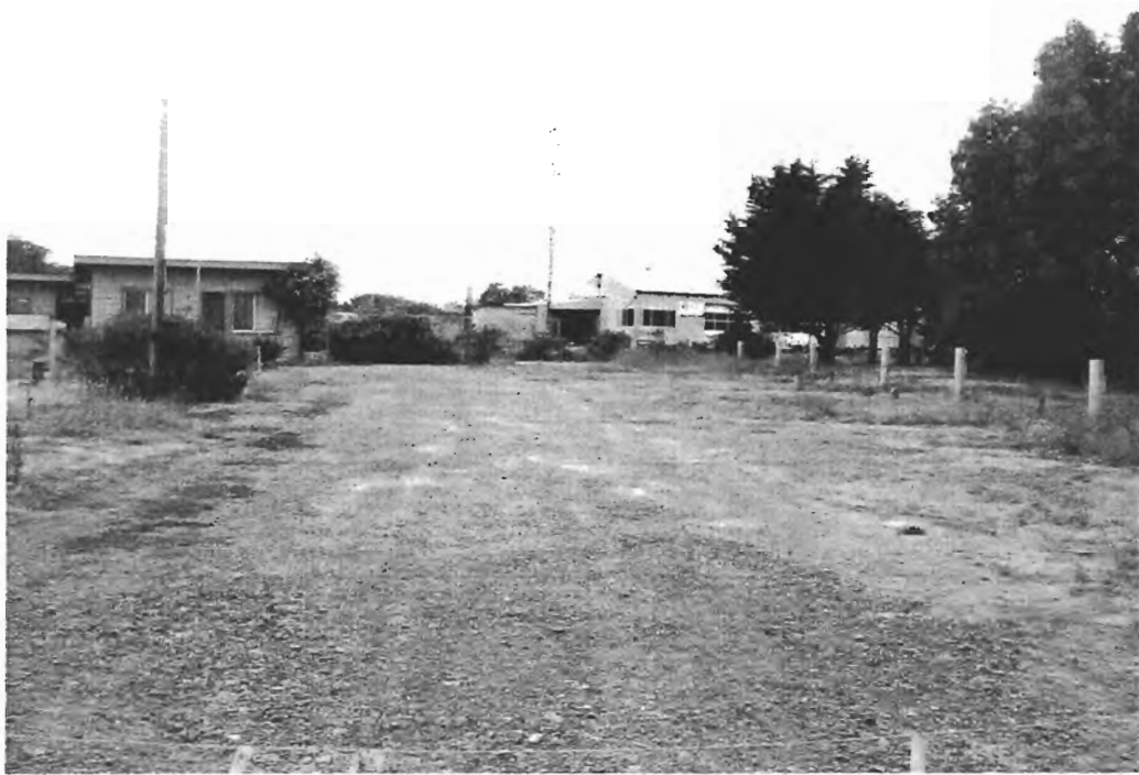
Existing Road Surface
