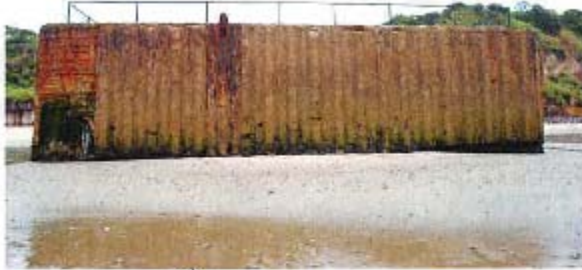
Photo 1 - PRC 421-2 Caisson Wall (looking north)
