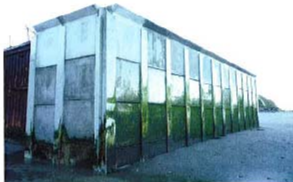
Photo 3 - PRC 421-2 Final Wall, (looking east)
