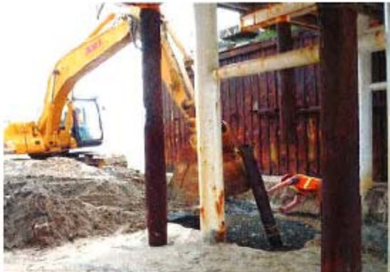
Photo 1 - PRC 421-2 Access Pier Pile Removal
