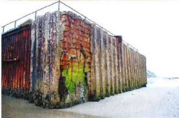
Photo 2 - PRC 421-2 Caisson Wall (looking northeast)
