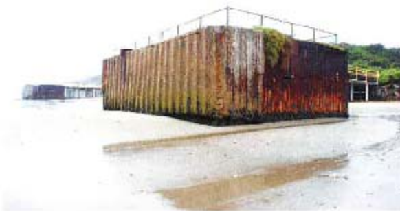
Photo 3 - PRC 421-2 Caisson Wall (looking west)
