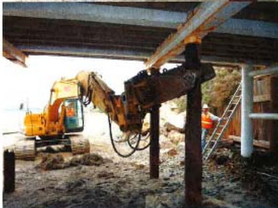
Photo 2 - PRC 421-1 Access Pier Cutting Pile
