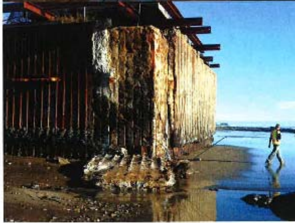
Photo 2 - PRC 421-2 Failed section of old wall necessitating 16th pile and panels
