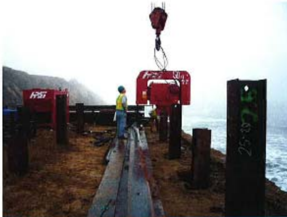
Photo 1 - PRC 421-2 False Work Piles with Vibrating Driver
