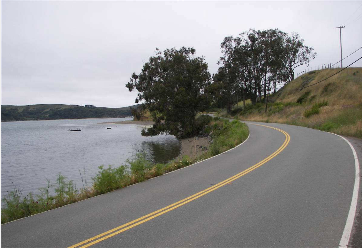
Photo 1. HWY 1 at Project Site, Facing Northwest
