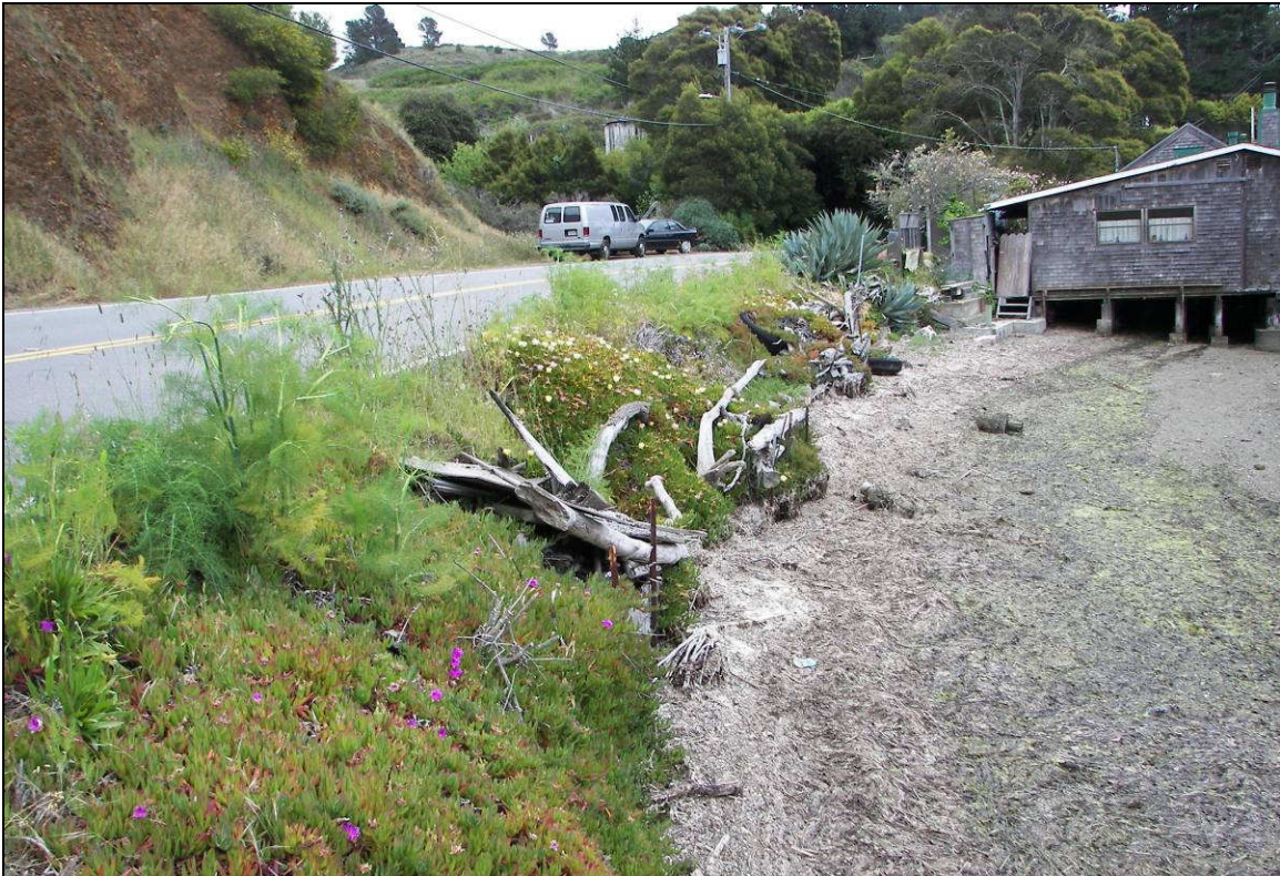
Photo 2. HWY 1 Embankment at the Project Site, Facing Southeast
