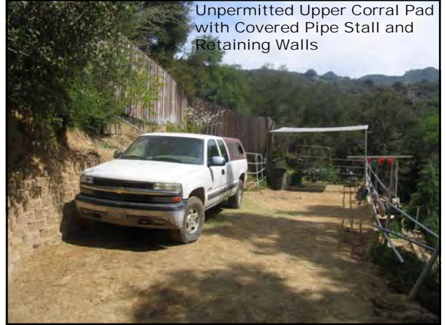
Unpermitted Road, Upper Corral Pad with Covered Pipe Stall, and Terraced Retaining Walls
