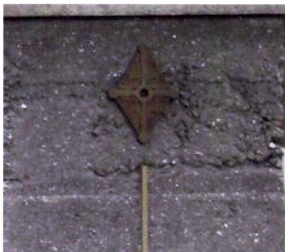
Concrete columns: Unpainted.
