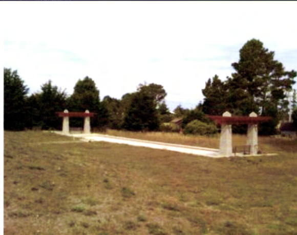
Bocce Court: Concrete columns with wooden trellis and low concrete perimeter enclosing a traditional oyster shell base.
