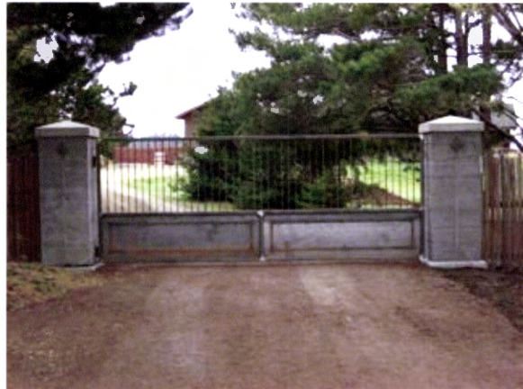
Entry Gate: Concrete columns with iron railing and steel kick plates.
