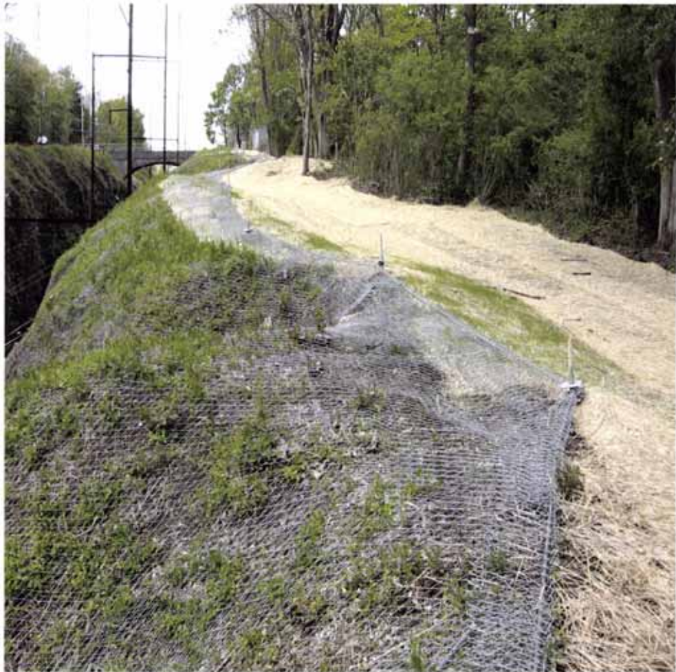
Gwynedd Pennsylvania Metal net staked along top of ridge and netting conforming to cliff side
