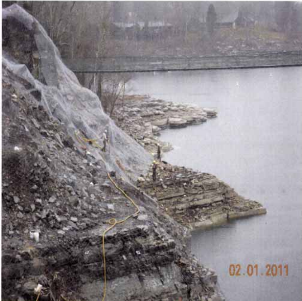
Daville Kentucky Draping and anchoring metal netting material over the rock cliff
