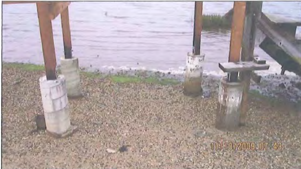
Pier footings at bayshore. Note small colony of Spartina upper right, unvegetated cobbled substrate, and sparse growth of Ulva along shoreline.
