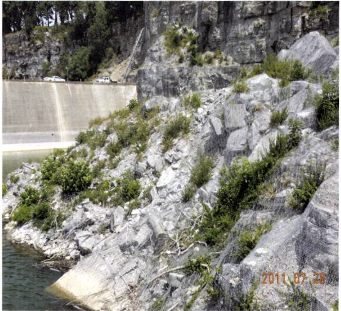
Daville Kentucky 6 months after installation vegetation is starting to grow through metal netting
