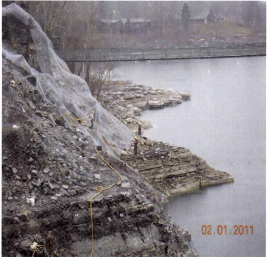
Daville Kentucky Draping and anchoring metal netting material over the rock cliff
