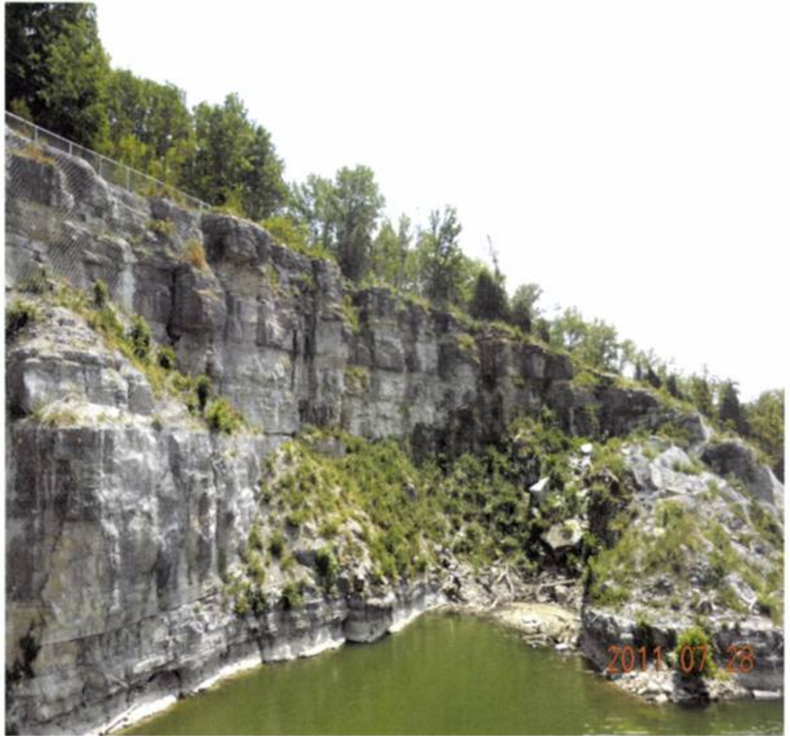
Daville Kentucky 6 months after installation, metal netting is practically invisible
