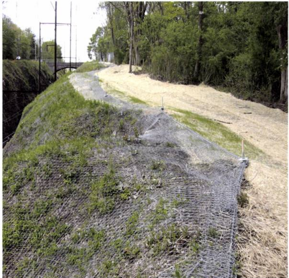
Gwynedd Pennsylvania Metal net staked along top of ridge and netting conforming to cliff side
