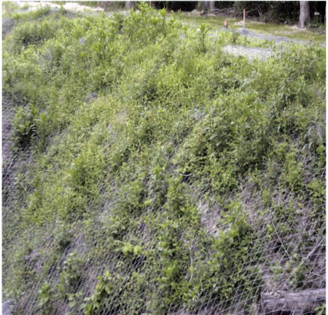
Gwynedd Pennsylvania Close up of vegetation growing through metal netting by June 2010
