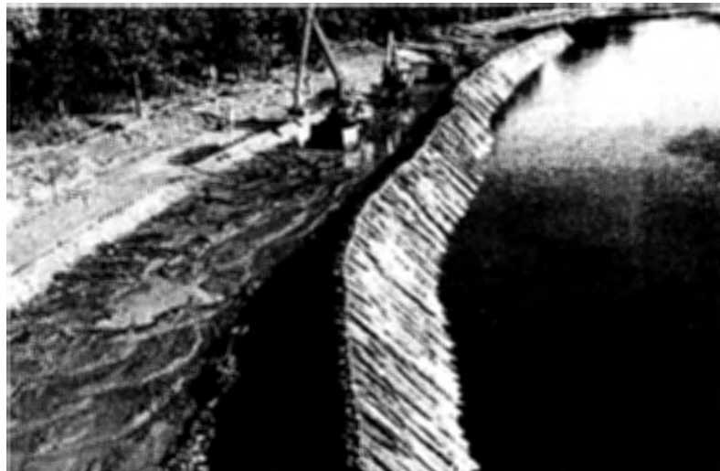
Placing membrane
