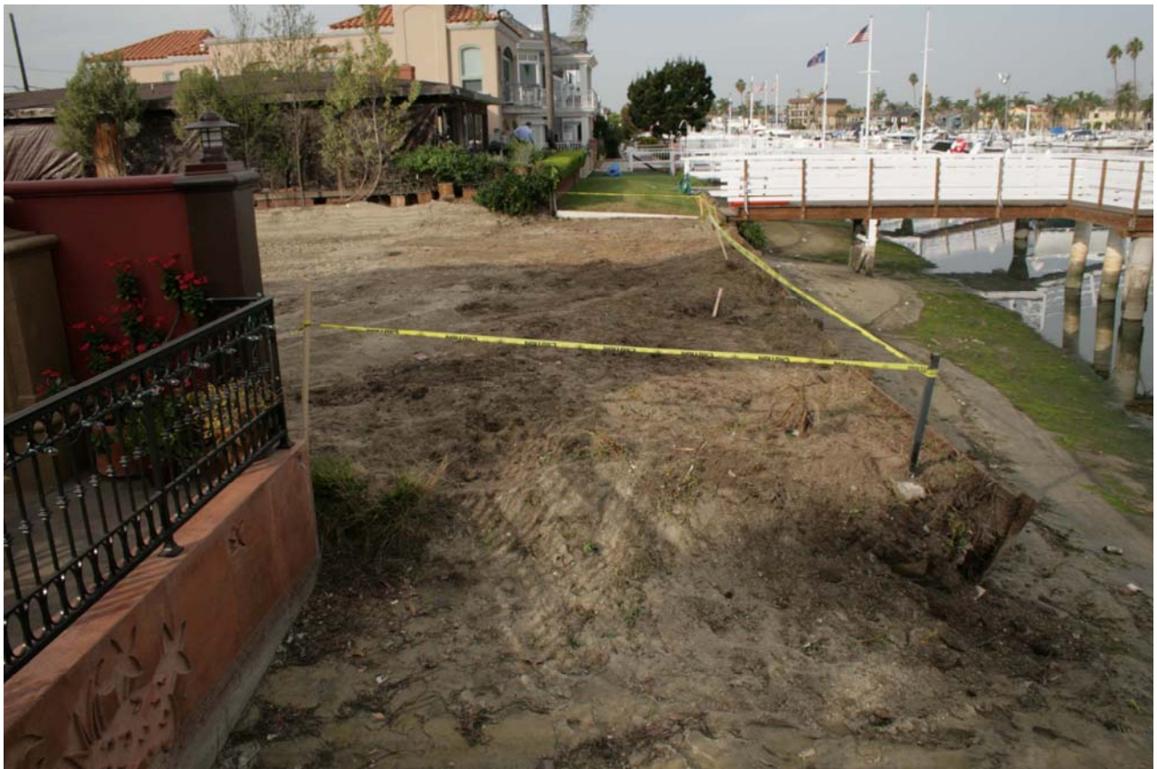
Yellow tape delineates the 15-foot wide public right-of-way at 5609 Sorrento Drive, Naples Island, CA (March 2012).
