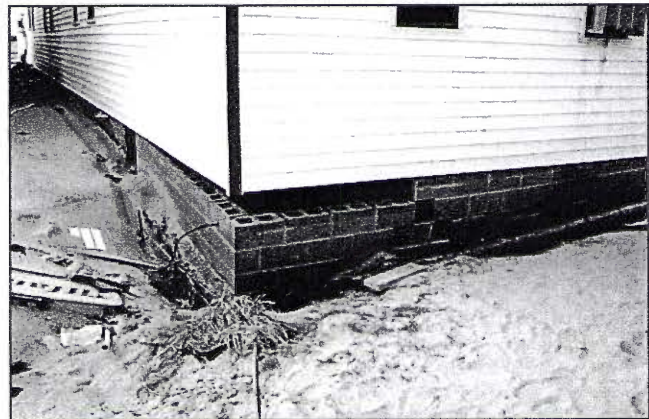
Failure of crawlspace foundation undermined by scour.
