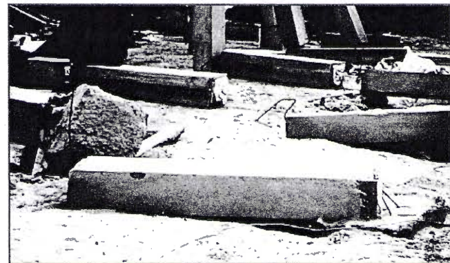
Pier (column) failures: footings undermined and columns separated from footings.
