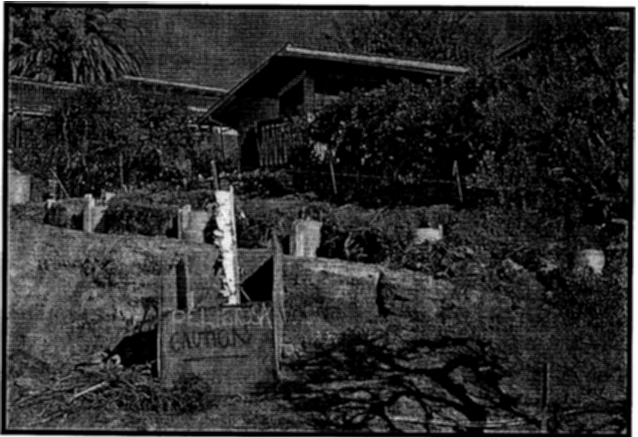
Photo 6 (soldier piles along east property line)
