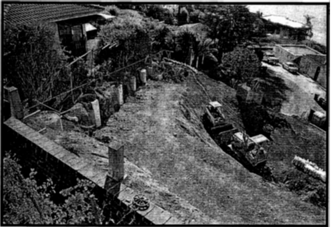
Photo 7 (soldier piles along east property line)
