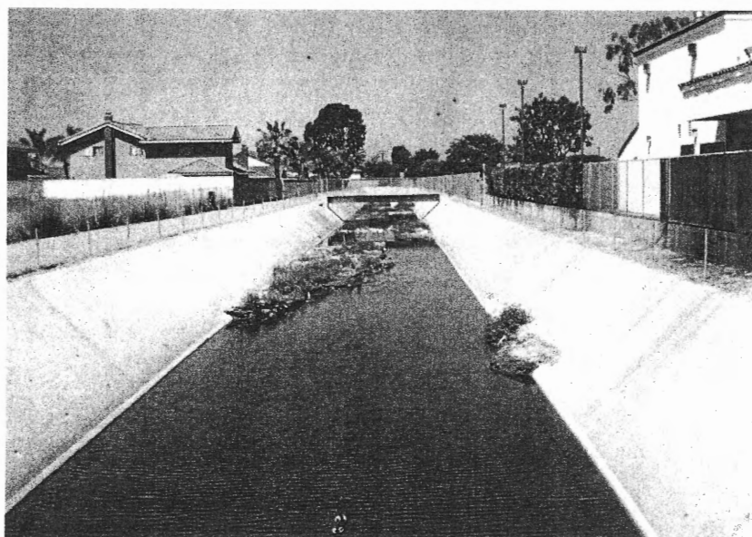
Representative trapezoidal channel with concrete sides and earthen bottom (Talbert Channel).
