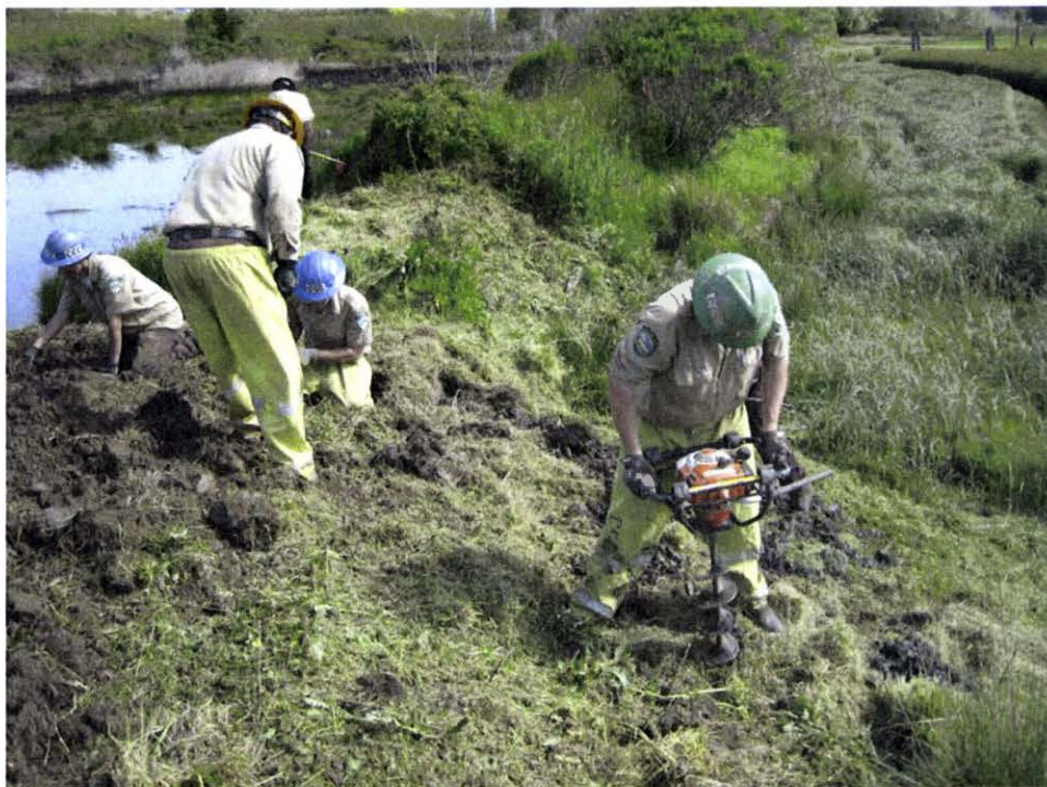
Figure 8. East side breaching by CCC crew (D. Allan, May 2011).
