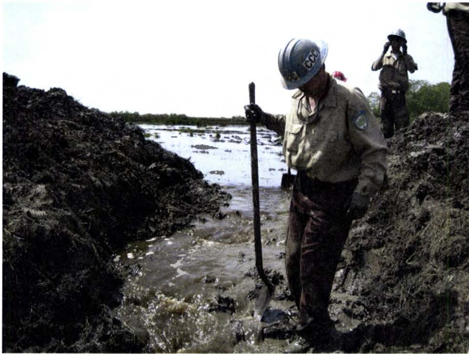
Figure 9. East side breach by CCC crew (D. Allan, May 2011).
