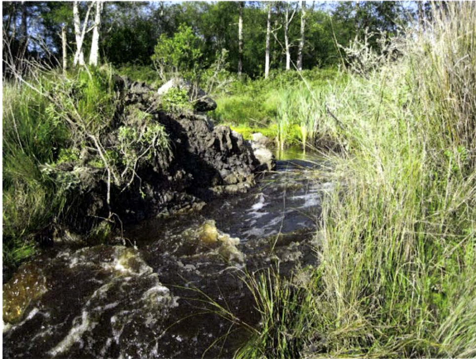
Figure 7. West-side dike breach by backhoe (D. Allan, May 2011).
