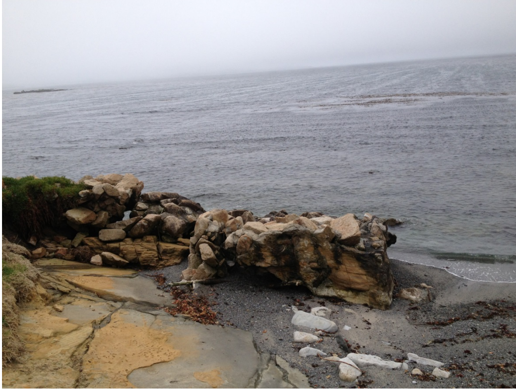
18 th Fairway Project Site Grouted Rip-Rap
