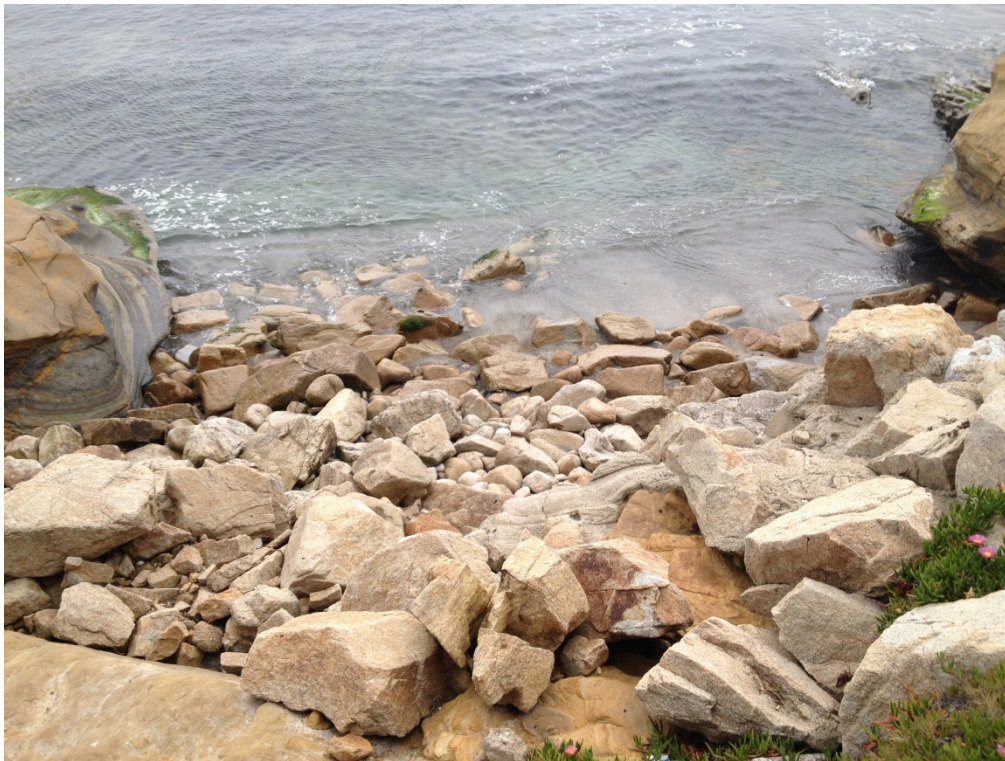
Sloat Project Site Concrete Rubble
