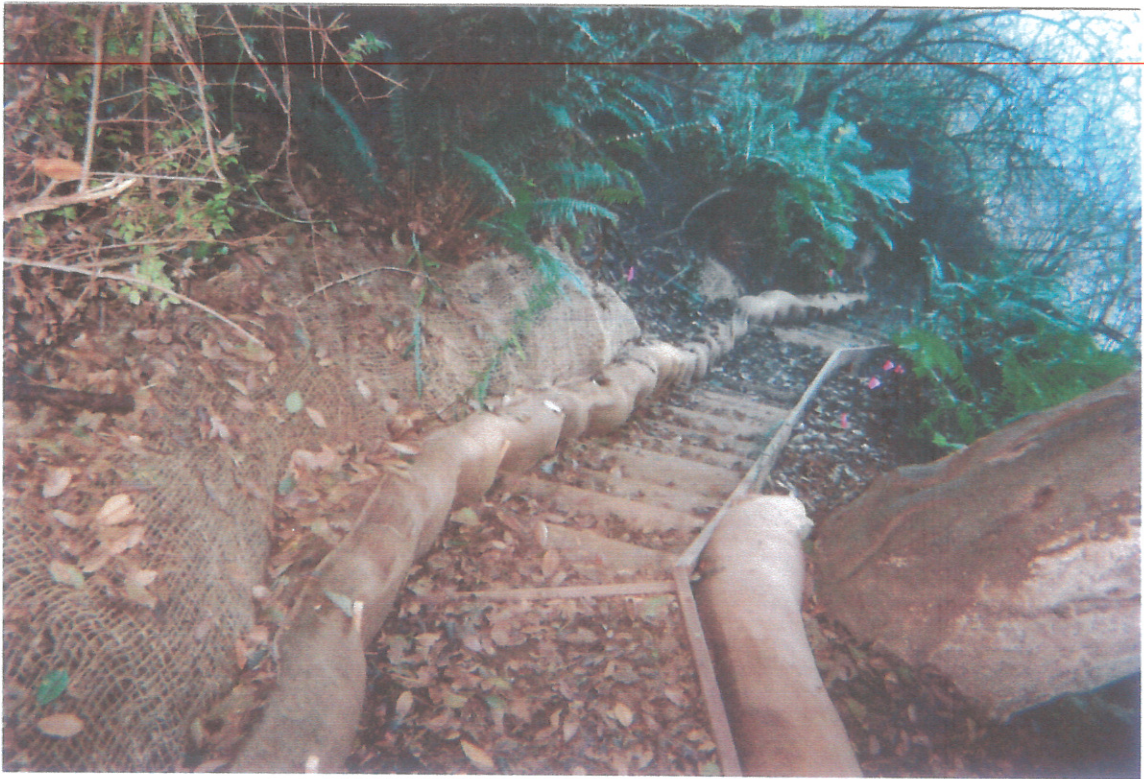
Stairs after installation of waddles.
