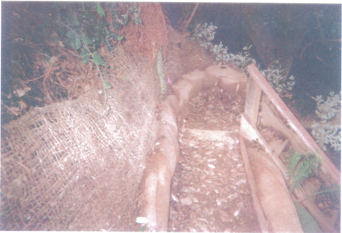
Stairs after installation of waddles.
