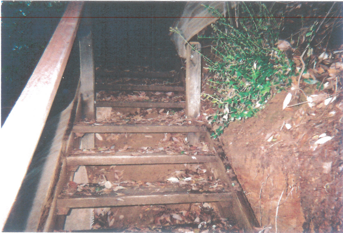
Stairs before installation of waddles. Note the 4 x 4 support posts on both sides, embedded into concrete piers.
