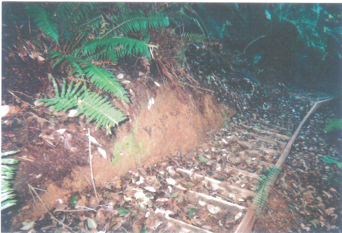
Stairs before installation of waddles. Note the 4 x 4 support posts on both sides, embedded into concrete piers.
