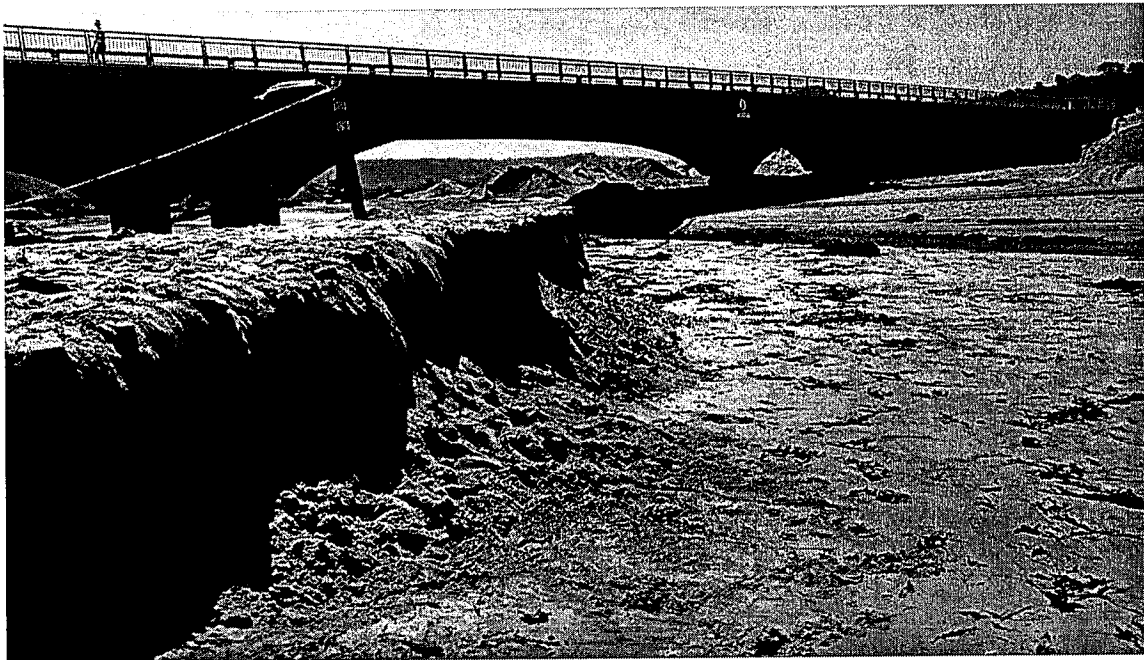
Figure 3. View of Beach Profile, Northern Edge of Los Peñasquitos Lagoon Inlet. May 15, 2013
