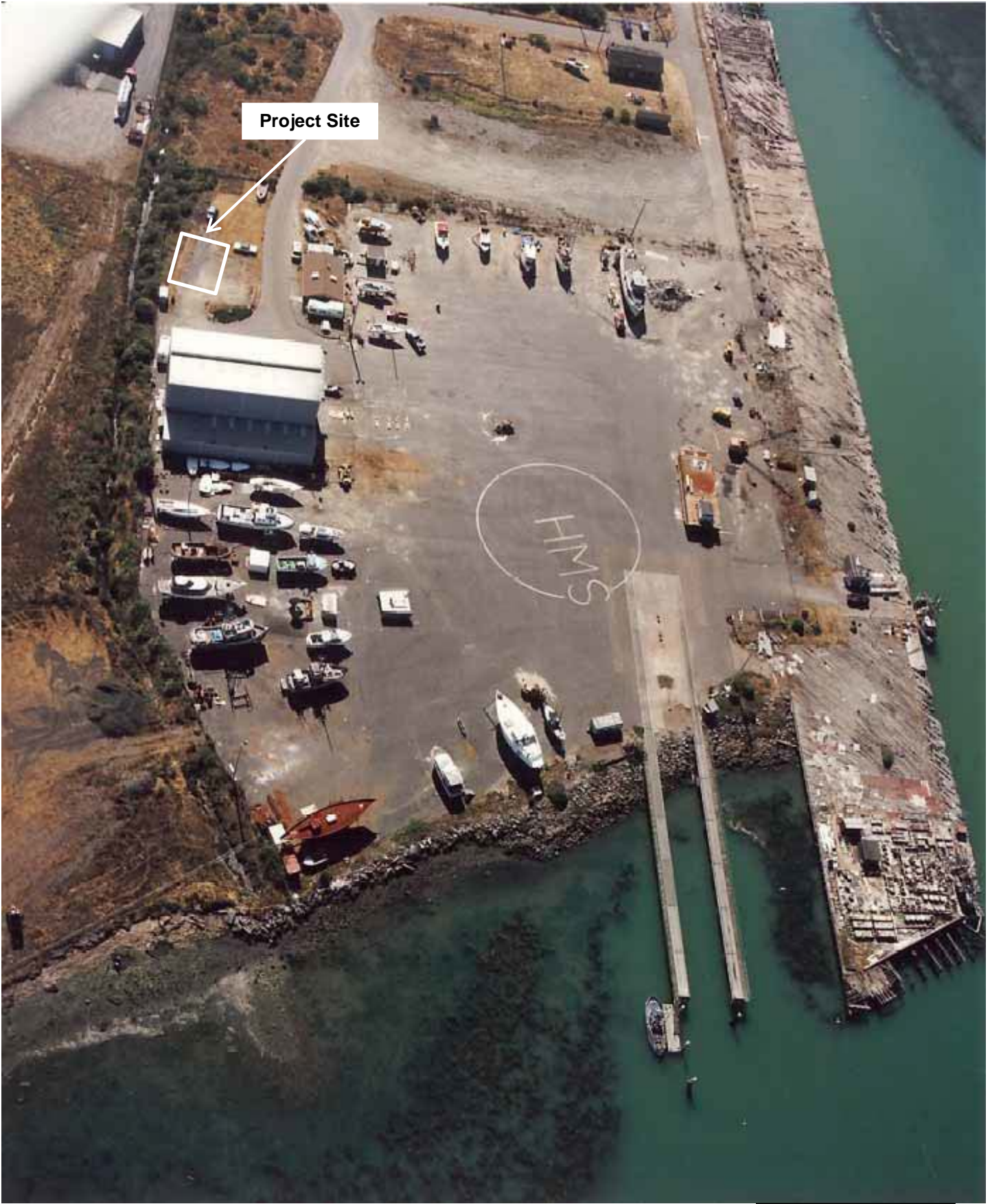
EXHIBIT NO. 4 APPLICATION NO. 1-12-022 T-MOBILE WEST LLC PROJECT SITE OBLIQUE AERIAL
