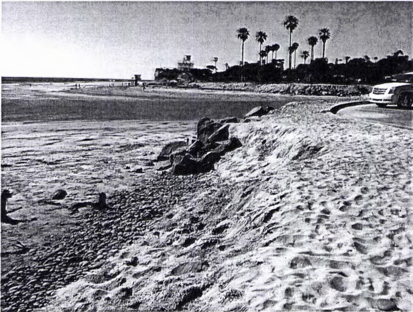
5/20/13 Beach View of Cardiff Reef Lot Turnaround Post-construction.
