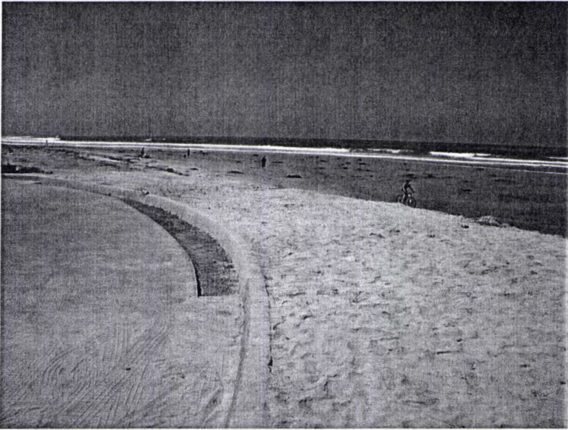
5/20/13 Shore View of Cardiff Reef Lot Turnaround Curb Replacement Post-construction.
