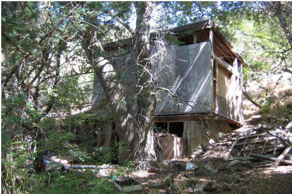
Existing 200sq. ft. structure proposed for removal
