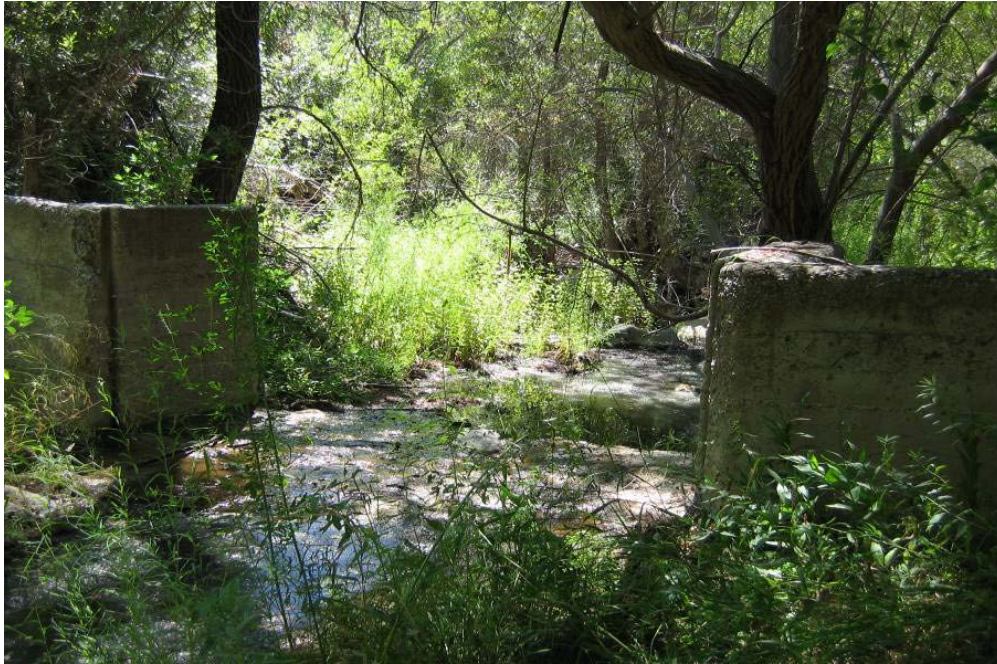
Existing Creek Dam abutments, prosed for removal
