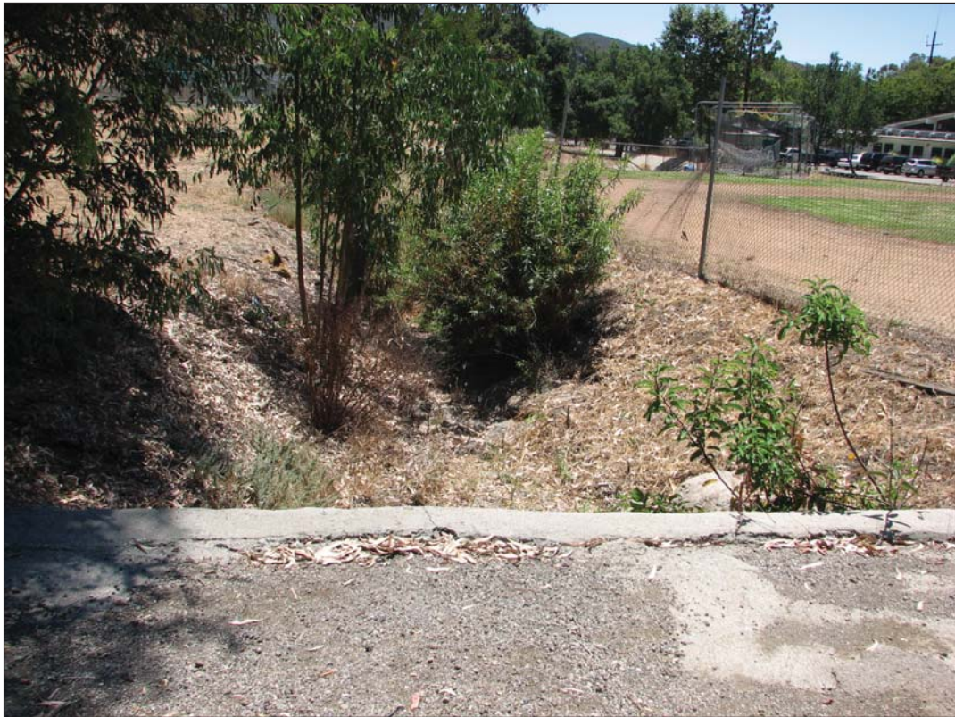
Eastern drainage: Looking south from a culvert at the drainage feature located just east of the ball field.
