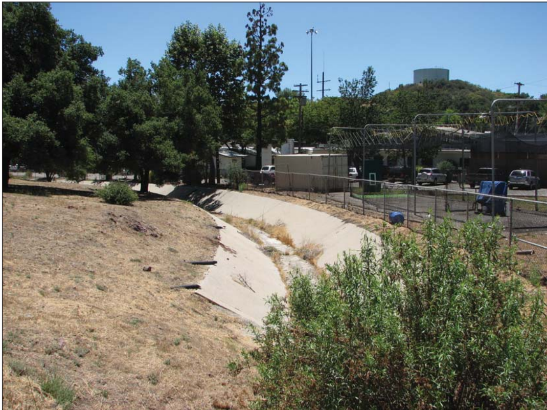
Culvert trap channel: Looking south from a culvert at the concrete trapezoidal channel adjacent to the ball field.
