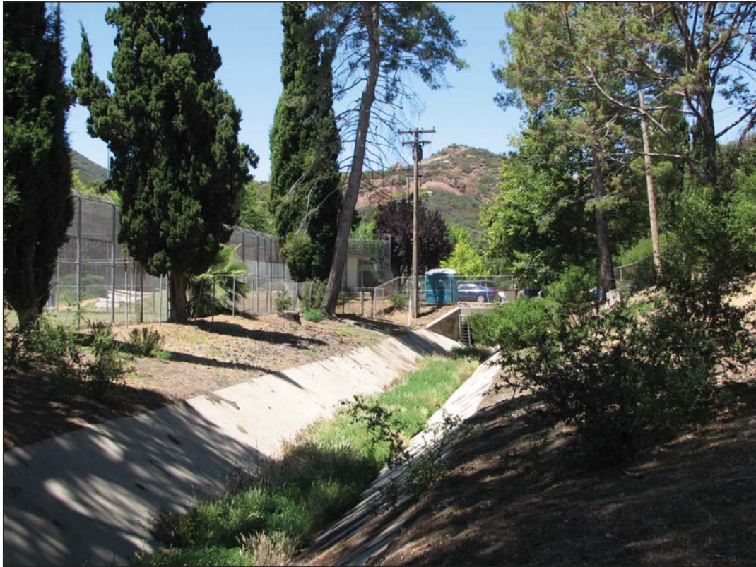
Just north of the Encinal Road and Miller Probation Camp Drive intersection.
