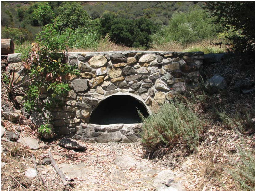
Culvert at eastern drainage: Looking north at a culvert/drainage feature located just east of the ball field.
