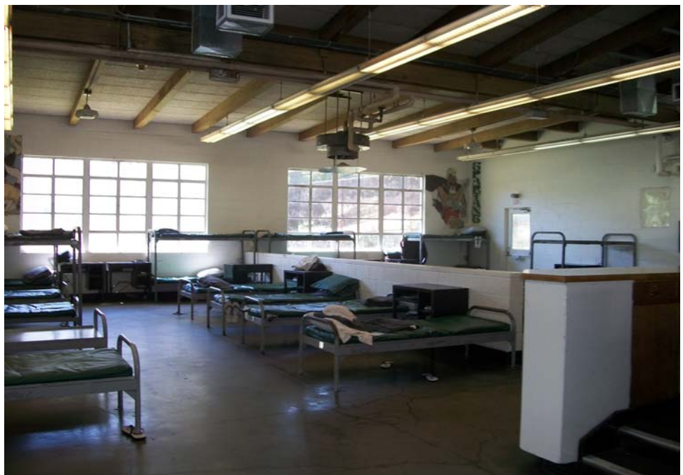
Photograph 6: View of the interior of a typical dorm structure.
