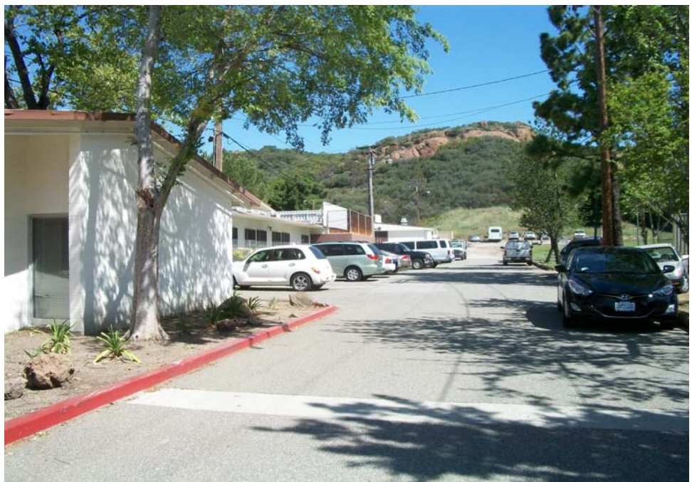
Photograph 2: View facing north of site buildings, parking areas, and driveways.
