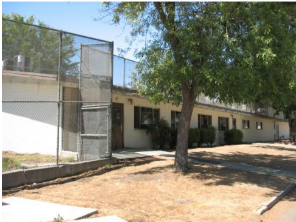
Photograph : Shared Kitchen and Mess Hall. View looking west.
